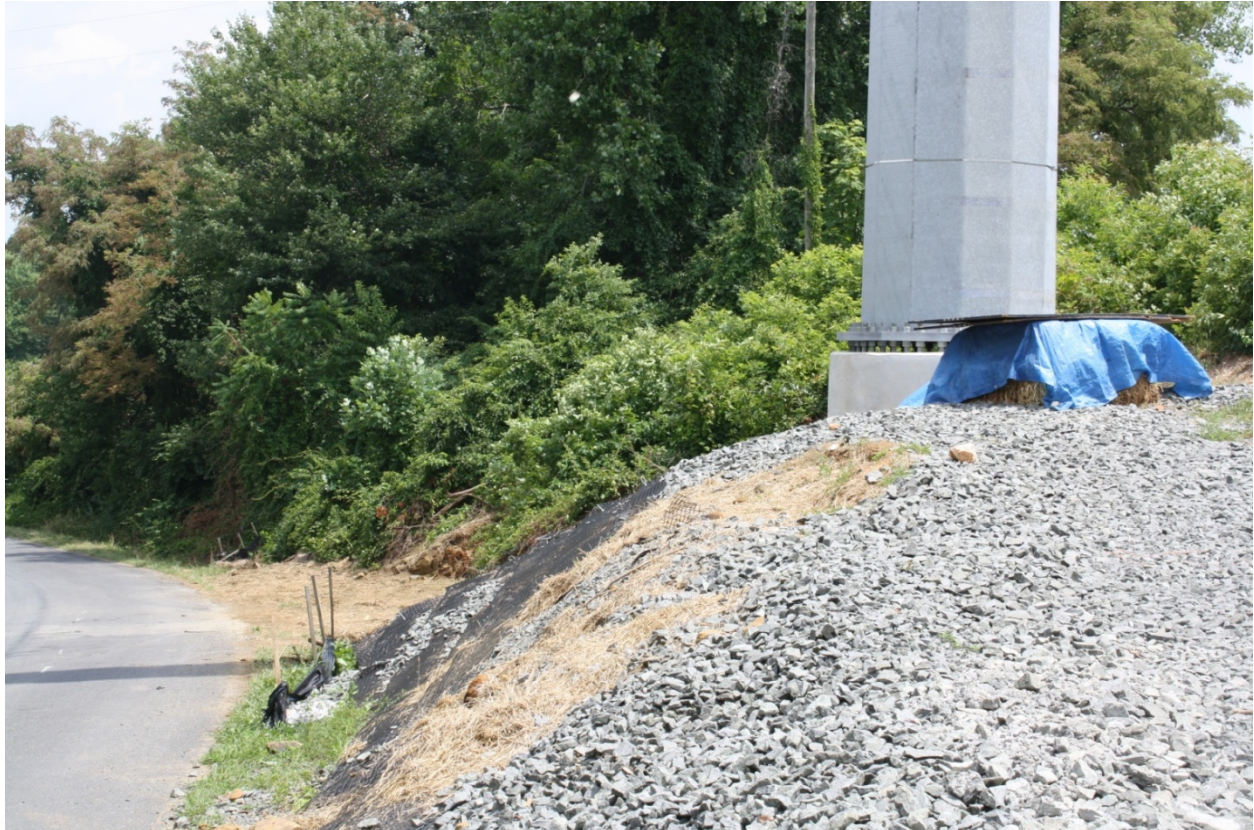
Figure 4.8 Dominion Transmission Pole located on VDOT ROW
