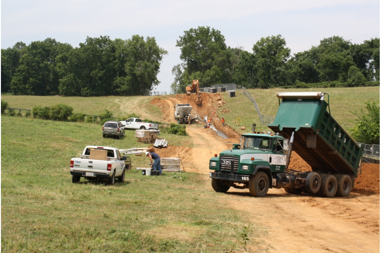
Figure 4.5 Laying of Underground HV Cable
