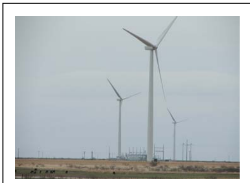
Figure 1.1 General Electric 1.5 MW turbine near Matador, TX
