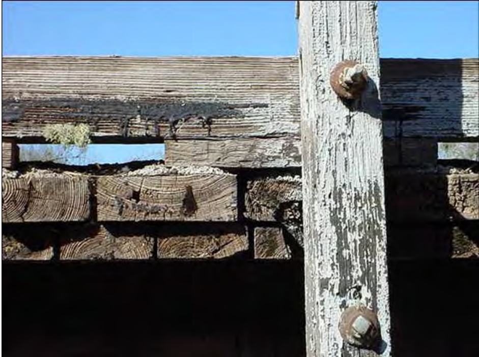
Coatings on wood posts or timber piles
