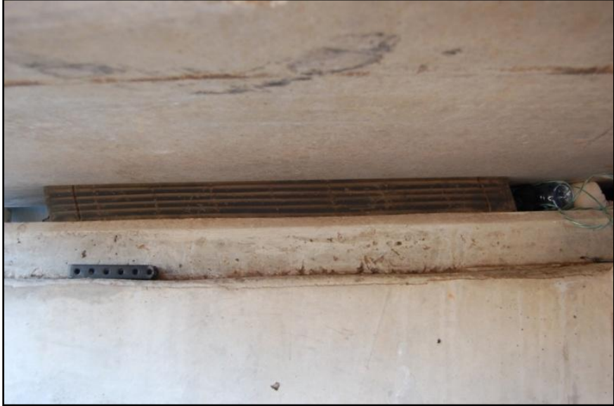
Figure 4.2 – Elevation of Bearing A
