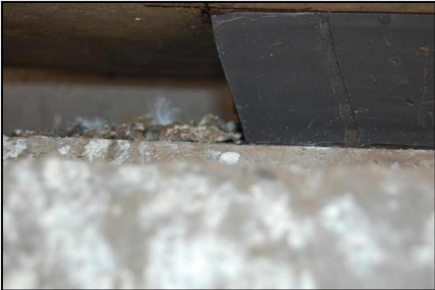
Figure 4.3 – Close-up of Bearing C
