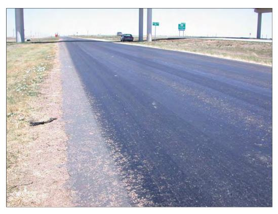
**Figure 3.2** Bleeding Asphalt Caused by Excessive, Heavy Truck Traffic and Hot Weather
