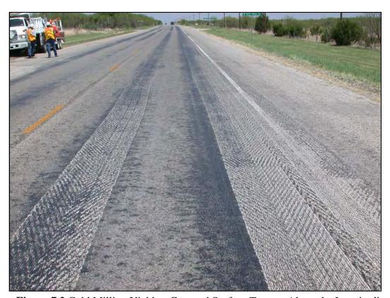
**Figure 7.2** Cold Milling Yields a Grooved Surface Texture Along the Longitudinal Axis of the Roadway
