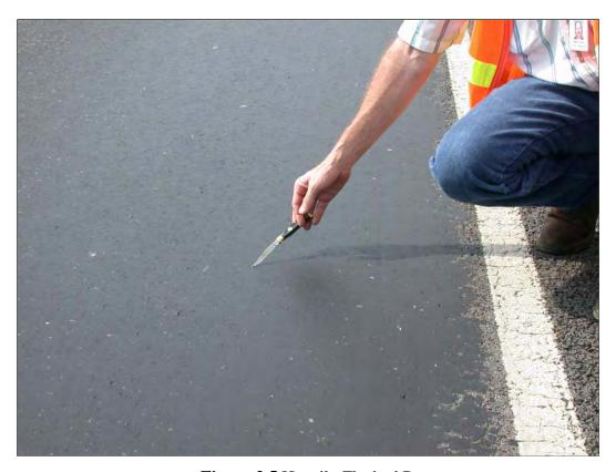
Figure 3.5 Heavily Flushed Pavement
