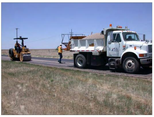
**Figure 6.3** Application of Grade 5 Aggregate to Treat Bleeding
