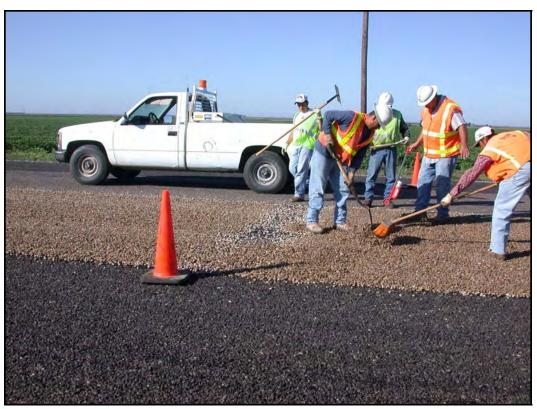
Figure 6.7 Hand Application of Aggregate to Treat Bleeding Pavement
