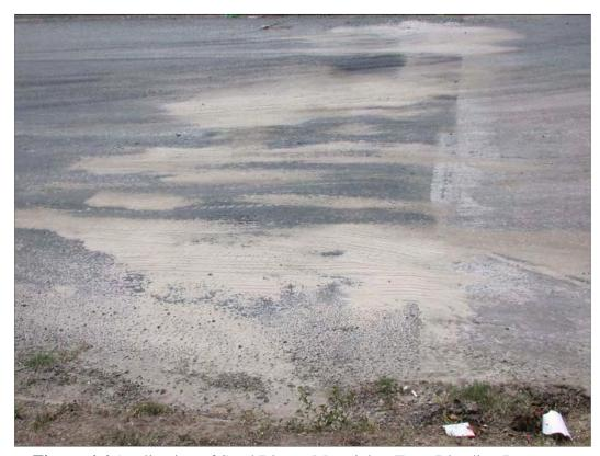
**Figure 6.6** Application of Sand Blotter Material to Treat Bleeding Pavement at an Intersection
