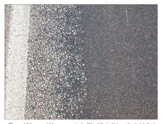
Figure 6.9 Improved Macrotexture in the Wheel Paths Using a Sandwich Seal
