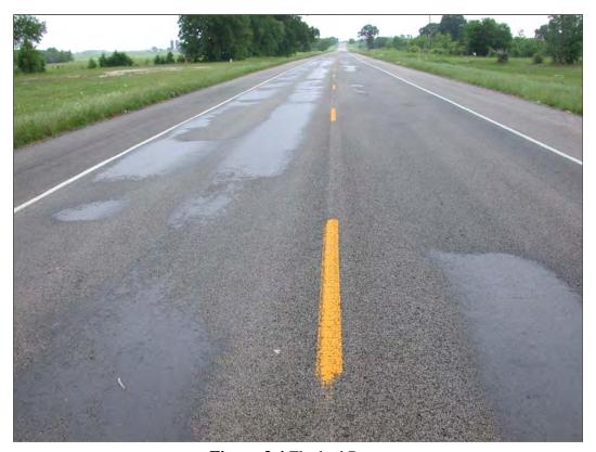
Figure 3.4 Flushed Pavement
