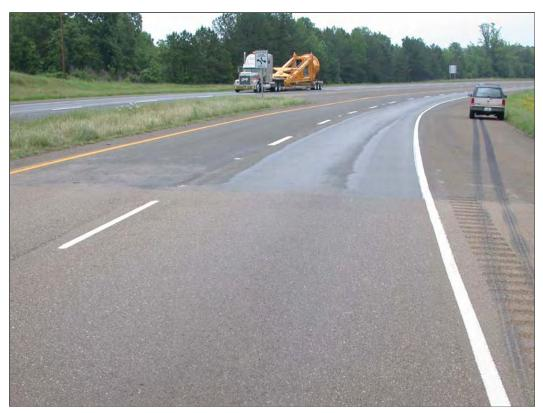
**Figure 7.7** Thin Overlays to Treat Flushed Pavement Can Be Applied Using Asphalt Laydown Machines
