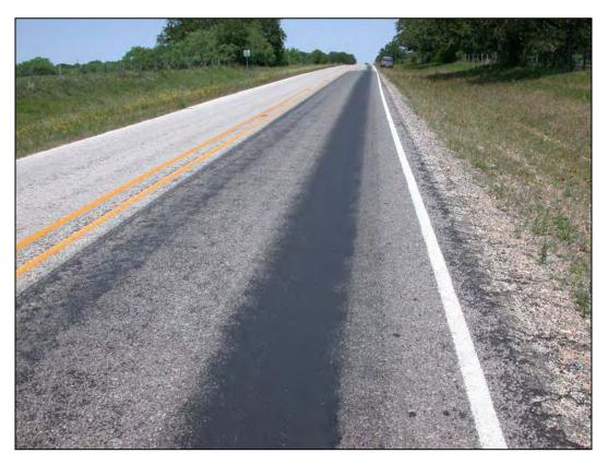
**Figure 4.1** Flushing in Wheel Paths
