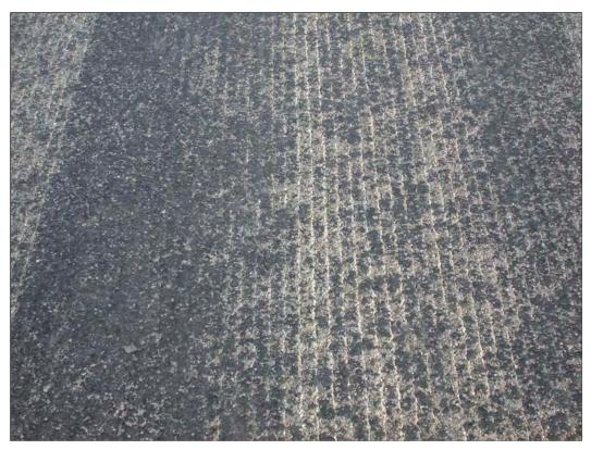
**Figure 7.10** Grooves in a Motor Grader Mold Board Can Score the Flushed Pavement to Improve Surface Texture
