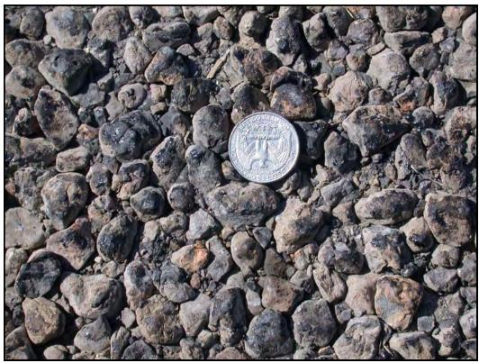
**Figure 8.3** The Racked-In Seal Involves a Light Application of Small Size Aggregate (Scatter Coat) Over a Traditional Coarser Aggregate Seal Coat
