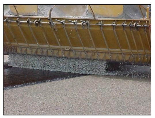
**Figure 6.5** Application of Grade 3 Seal Coat Aggregate
