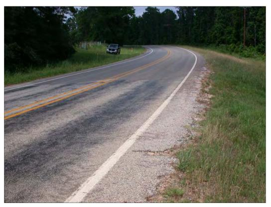
**Figure 7.6** Blade Level-ups and Other Thin Asphaltic Concrete Overlays Restore Friction and Skid Resistance
