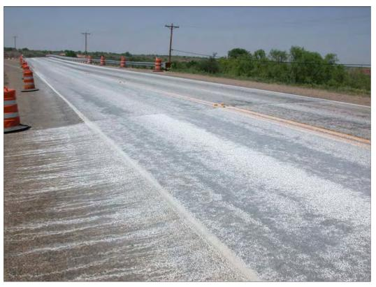
**Figure 6.12** The Lime Application Rate Should Achieve Good Splatter (Dosage) of Lime Water Solution on the Affected Pavement Surface
