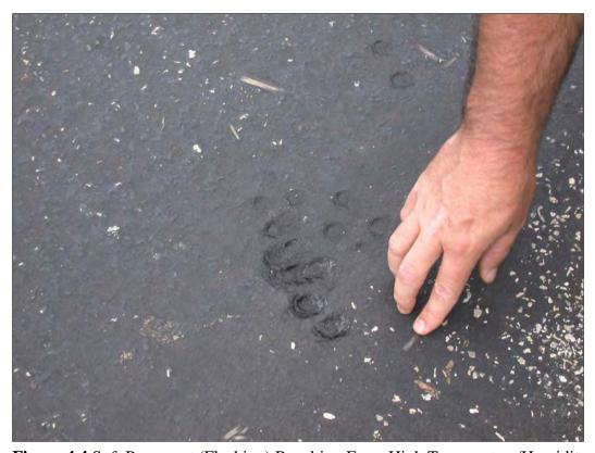
Figure 4.4 Soft Pavement (Flushing) Resulting From High Temperature/Humidity
