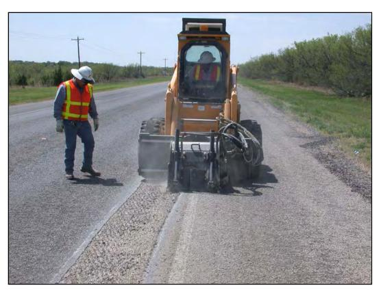
**Figure 7.1** Cold Milling to Retexture Flushed Pavement in the Wheel Paths
