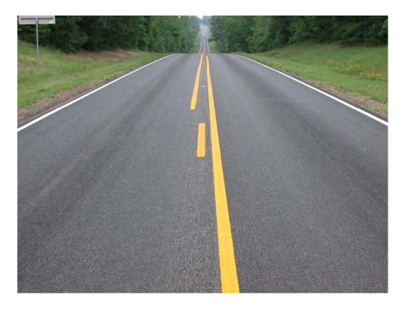
**Figure 7.4** Microsurfacing Can Be Used to Remediate Minor Rutting, Flushed Pavement, Poor Ride Quality and Low Skid Resistance
