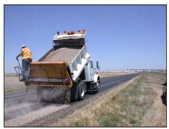
Figure 6.1 Applying Small-Size Aggregate to Treat Bleeding Pavement
