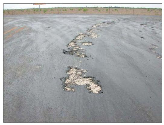
Figure 3.3 Pavement Damage – Picking Up of Seal Coat – Caused by Bleeding
