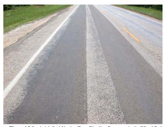
Figure 6.8 Sandwich Seal Used to Treat Bleeding Pavement in the Wheel Paths
