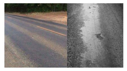
(a) (b) Figure 4.15 (a) Flushing and (b) Bleeding in Asphalt Surface Treatments
