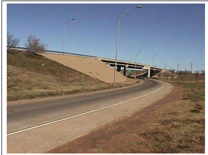
Figure 4.1 Side View of Riprap with Washed-Out Fines at Toe
