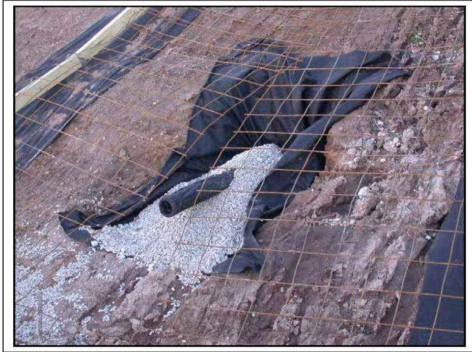
Figure 4.6 Filter Fabric at Drain in Riprap Slab during Construction
