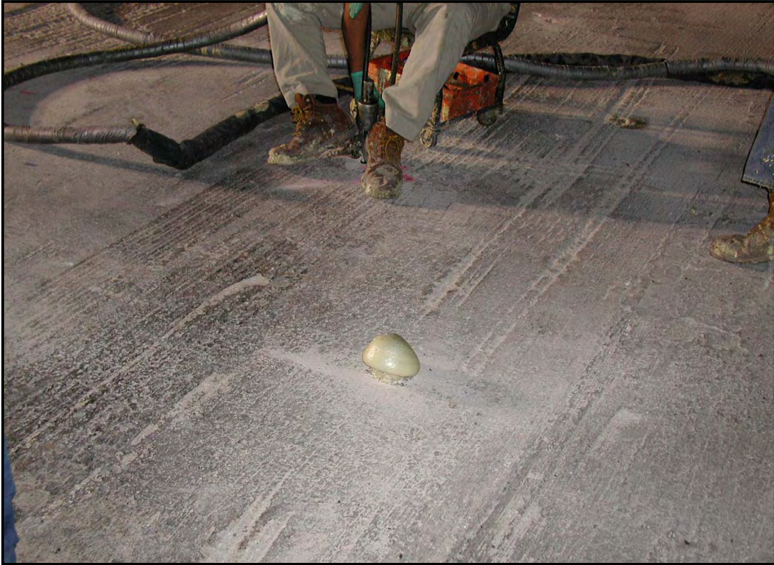
Figure 5.18 URETEK Slab Jacking Process
