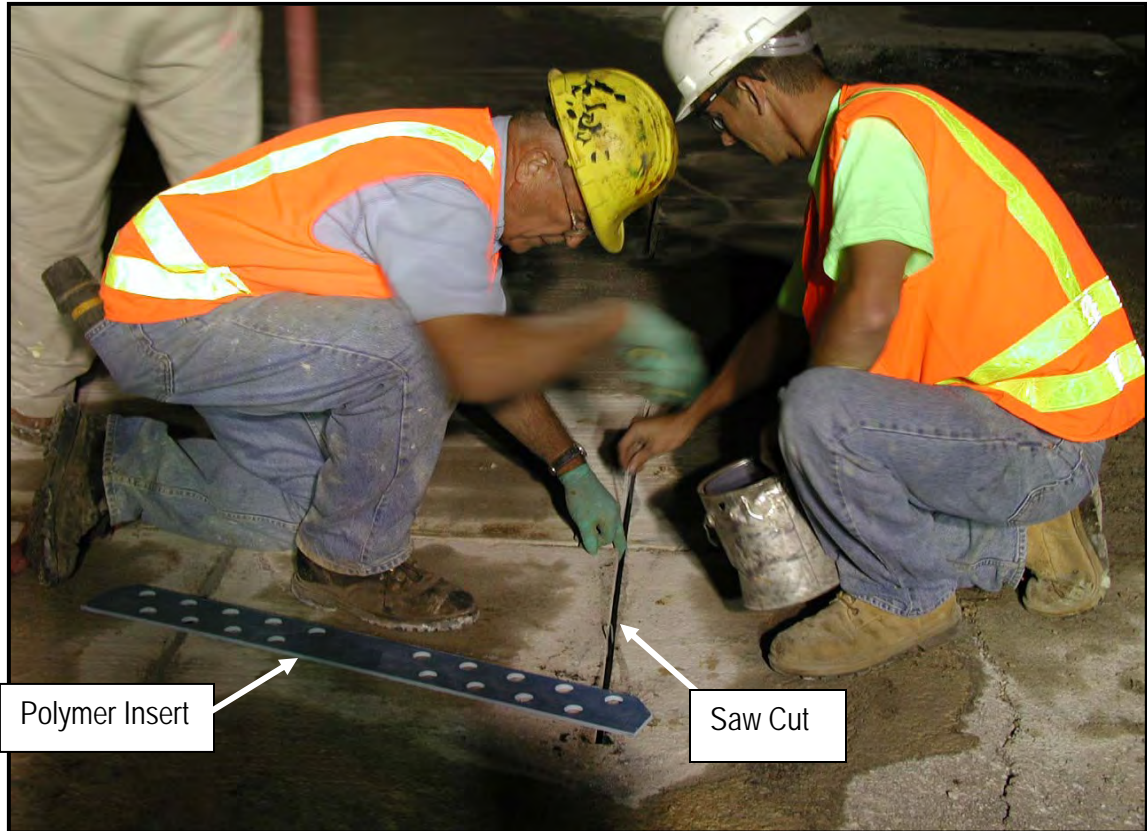
Figure 5.21 Sawcut Prepared to Receive Polymer Insert
