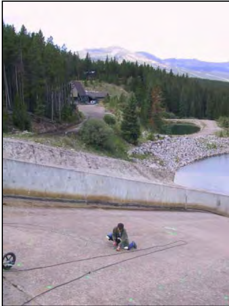
Figure 5.13 GPR and Slab-IR Testing of Alpine Dam Spillway to Detect Voids Underneath Slab ( Source: Olson Engineering Inc. )
