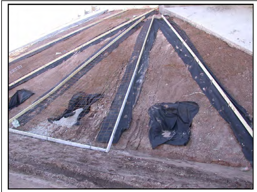
Figure 4.5 Filter Fabric at Joint in Riprap Slab during Construction
