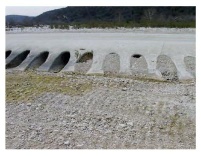
Figure 2.2: RR 335 at Ben Williams Ranch crossing Nueces River about 12 miles northeast from Barksdale, Edwards County, Texas. (Near the Real County line). Upstream side near river. All culverts have gravel deposit except for the southern four culverts which currently (03-09-2003) are passing flow. The other culverts also pass some flow, but behave as porous medium.
