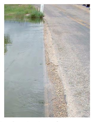
Figure 2.4: US 374 Northwest from Telegraph, Texas (between Junction and Rocksprings, Texas). Image is on a tributary of the South Llano River. Notice the vortices near the front left of the image at the water-roadway interface.
