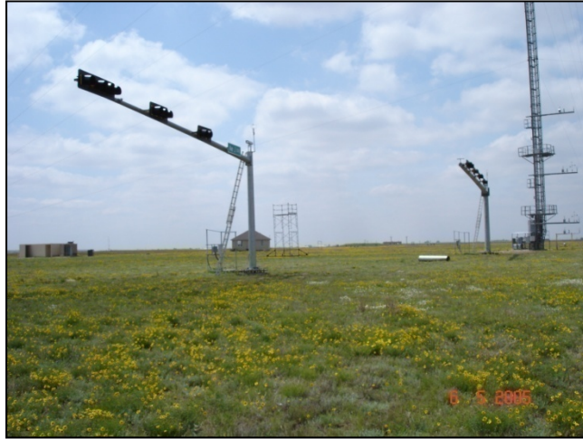
Figure 1. Two Cantilever Traffic Signal Structures Tested at Reese Technology Center
