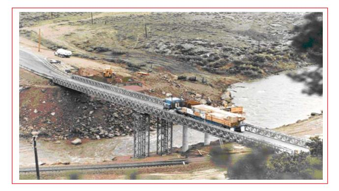
Figure 2. Acrow Temporary Truss Panel Bridge and Supports (Provided by Acrow Corp.)
