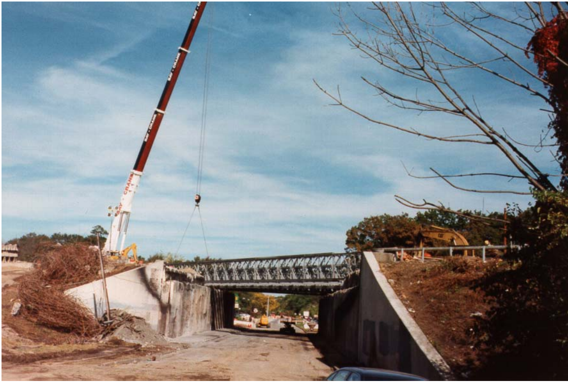
Figure 4 Two temporary bridges in Yonkers (provided by NY State Thruway Authority)
