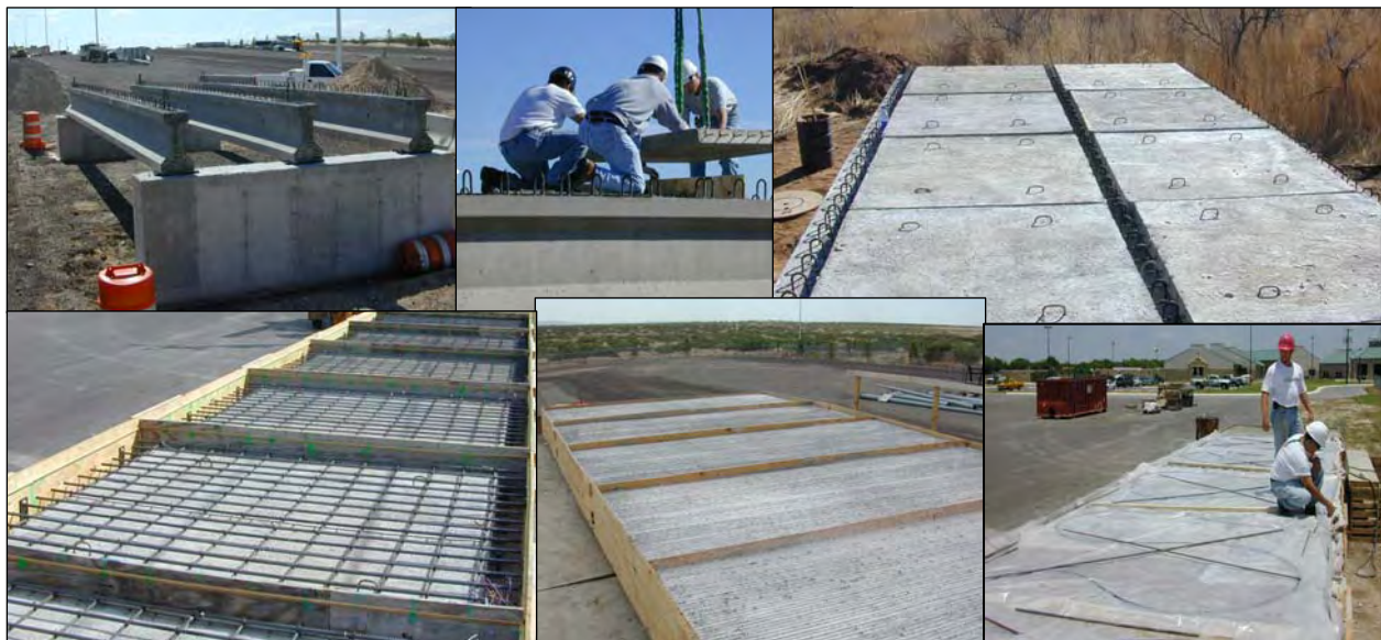
Figure 1. Construction of a Two-Bay Model Bridge Deck Slab
