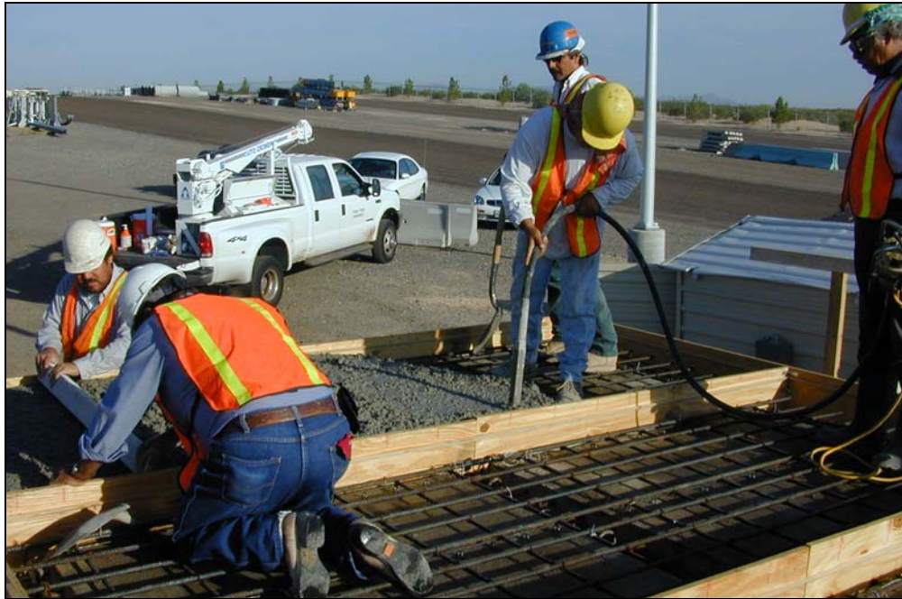
Figure 2.9 Placement of Concrete
