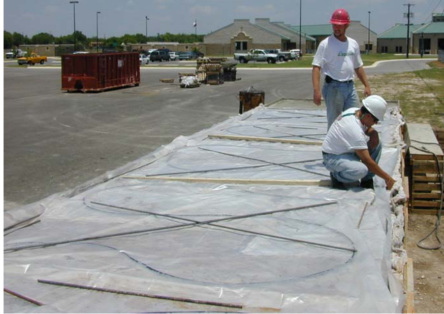
Figure 2.11 Finished Bridge Deck with Curing Media
