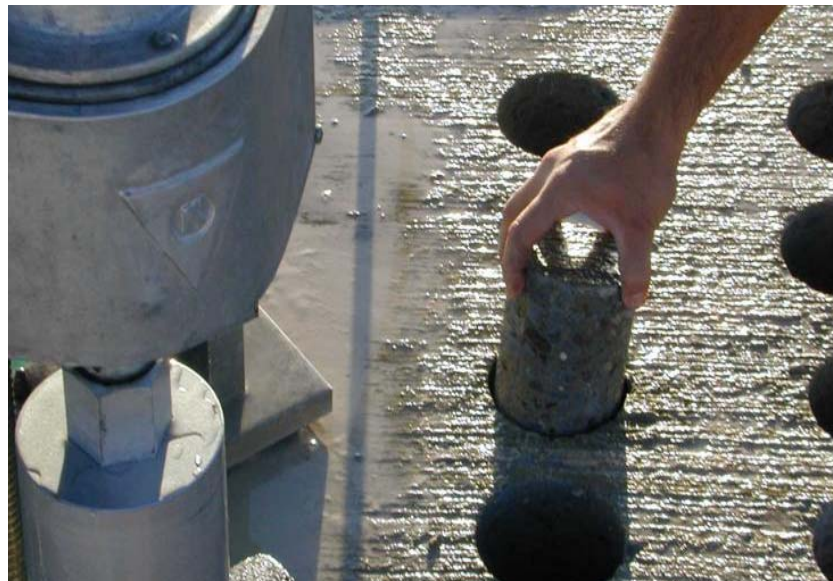
Figure 2.19 Four-Inch Concrete Core Being Retracted
