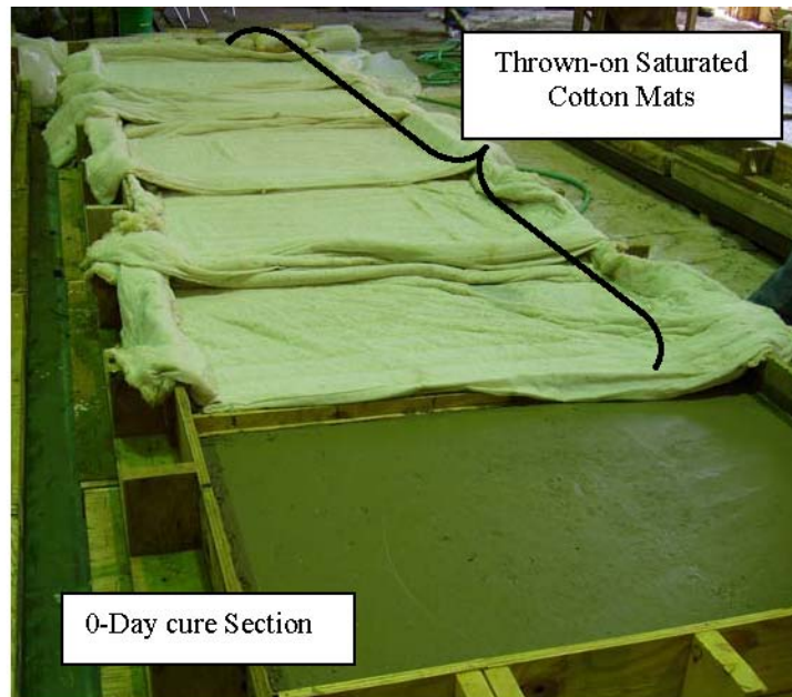
Figure 4.8 “Throw-on” Cure Slab with Saturated Cotton Mats
