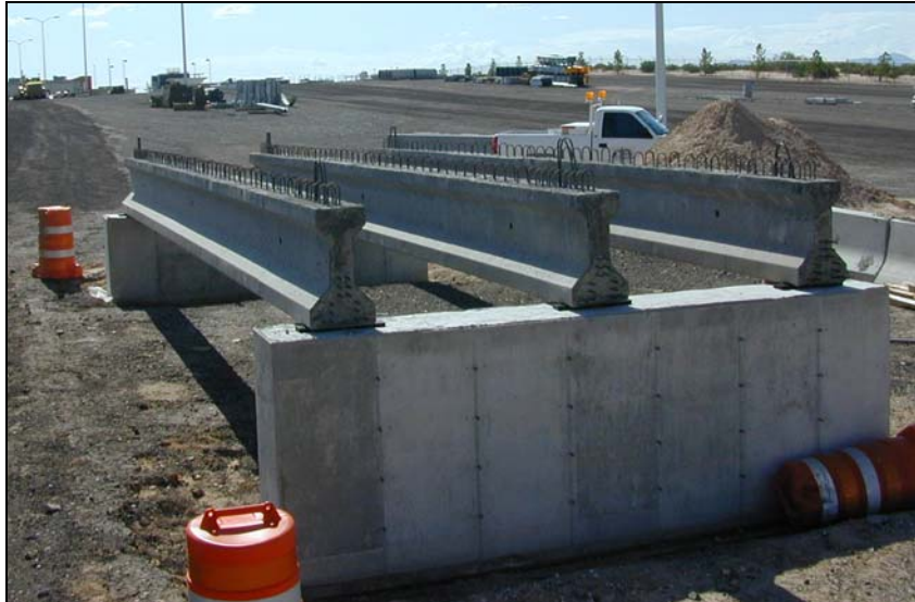
Figure 2.3 Placed Concrete Beams on Abutment Walls
