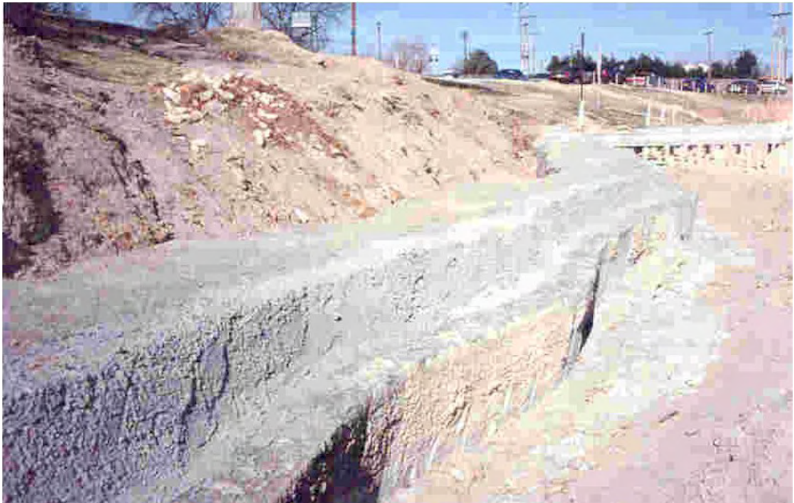
Figure 5.10 Partially Completed Retaining Wall Containing Tire Bales (NMED 1999)
