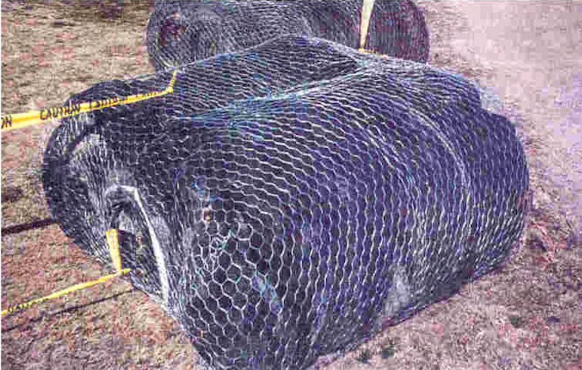
Figure 5.7 Bale Wrapped in Wire Mesh Before Encapsulation in Cement (NMED 1999)
