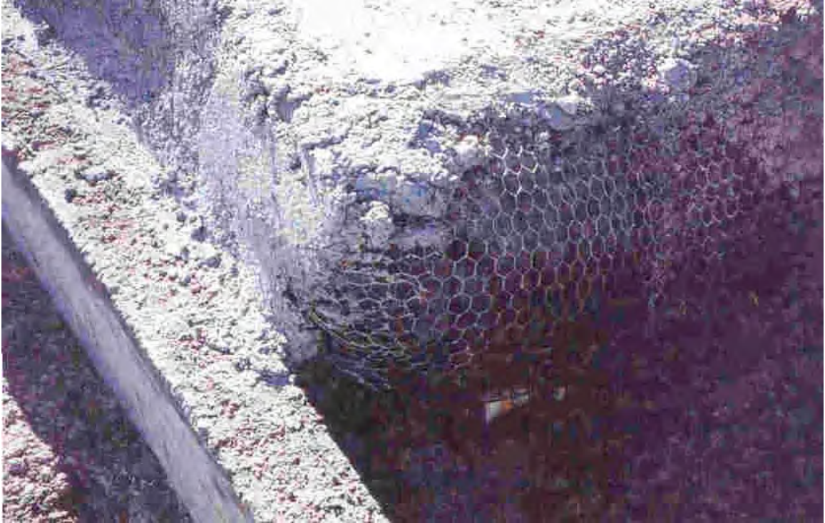
Figure 5.9 A Tire Bale Partly Encapsulated in Cement (NMED 1999)
