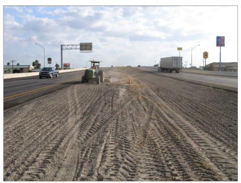
Figure 1.1. Seeding a Recently Completed Right of Way along US HWY 77 in South Texas.
