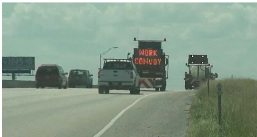
Figure 23. Work Convoy Vehicles during Mobile Operations.
