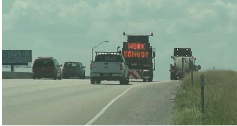
Figure 28. Work Convoy Vehicles during Mobile Operations.
