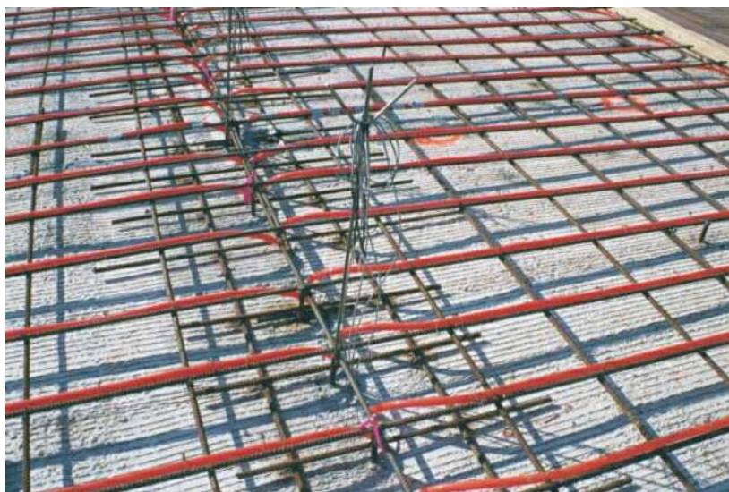
Figure 13-6. Bridge Deck Showing Instrument Wire on Trees.
