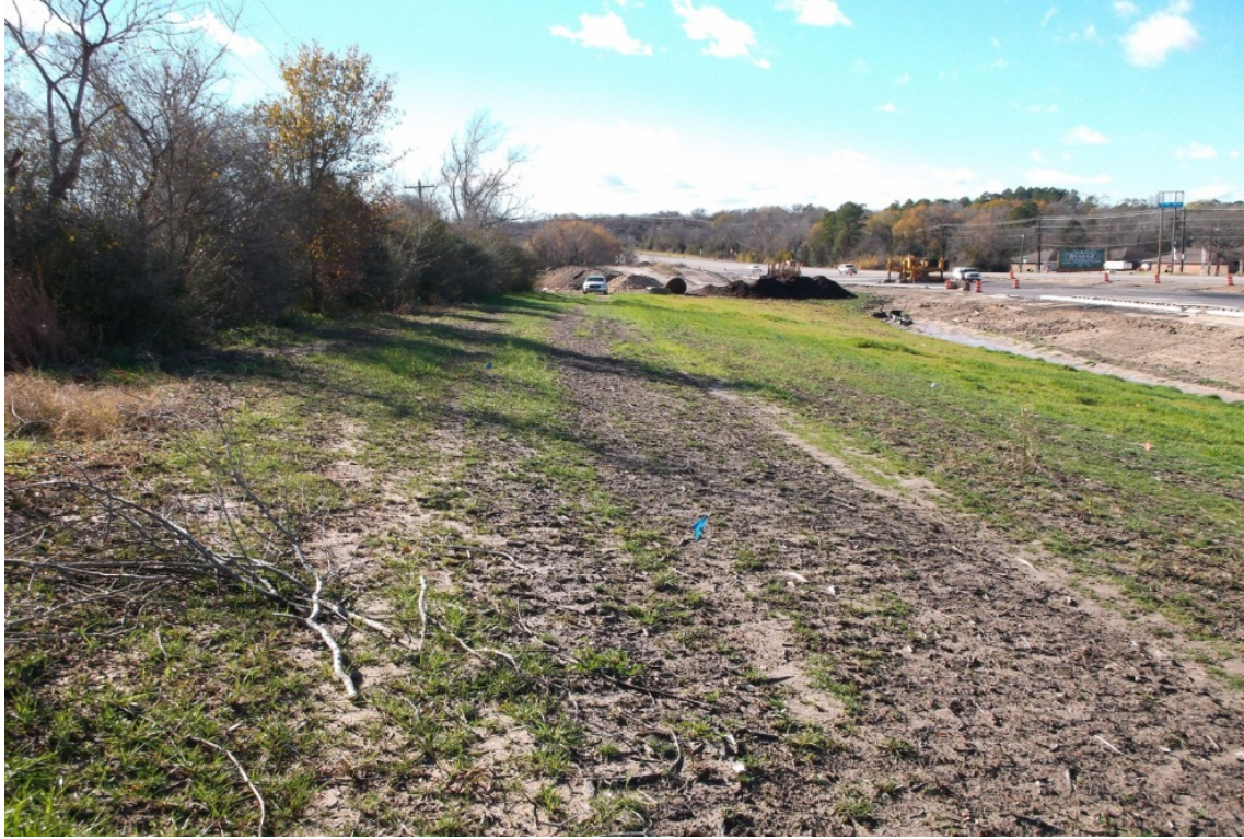
Figure 31. Prepared site at Bryan, Texas in October 2012.
