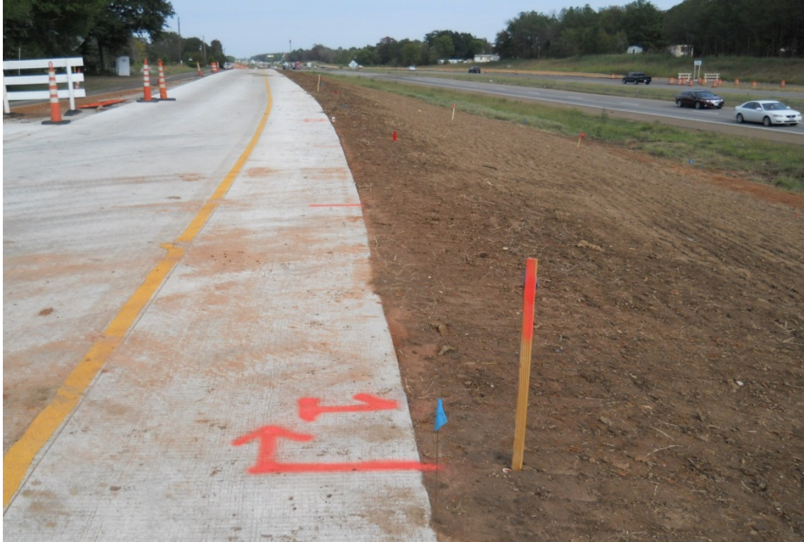
Figure 25. Prepared site at Hooks, Texas in October 2012.
