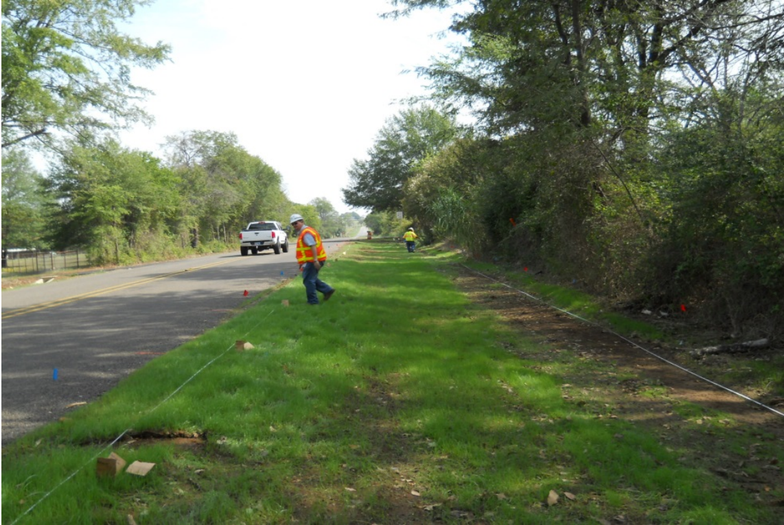
Figure 27. Prepared site at Grand Saline, Texas in October 2012.
