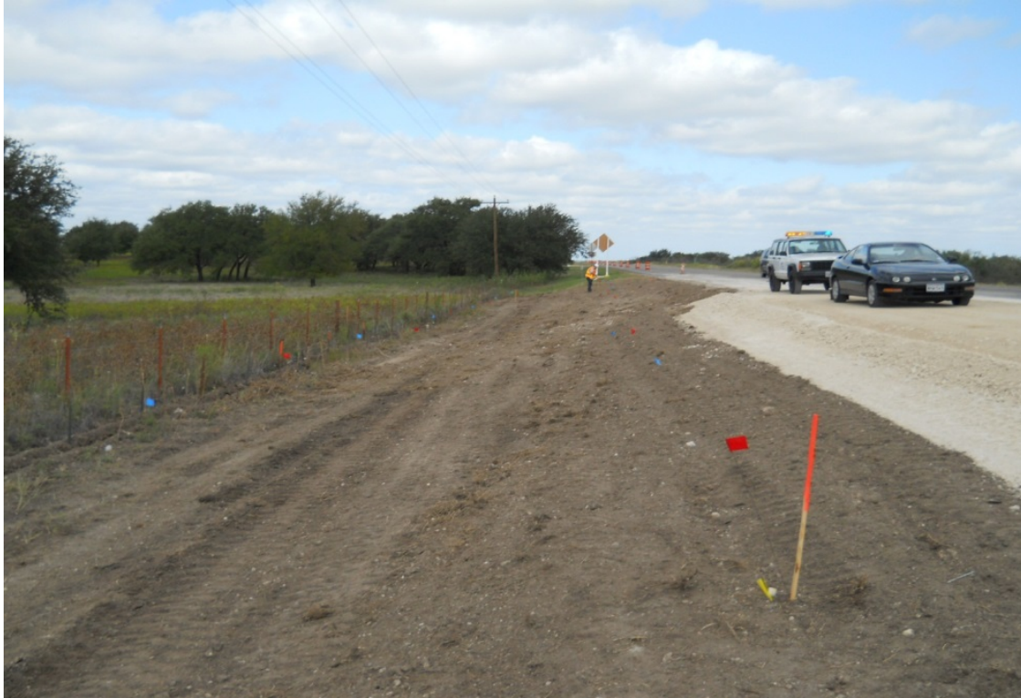
Figure 29. Prepared site at Zephyr, Texas in October 2012.
