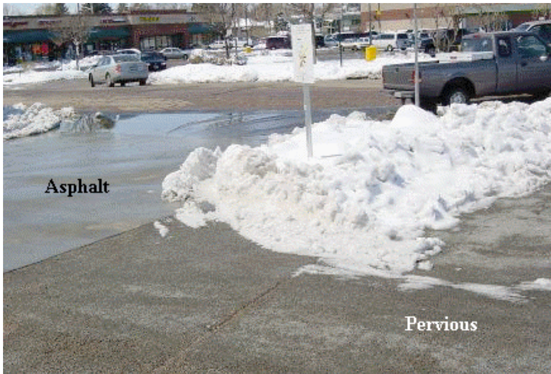
Figure C.10: Difference between asphalt and pervious concrete roads (National Ready Mixed Concrete Association 2006).
