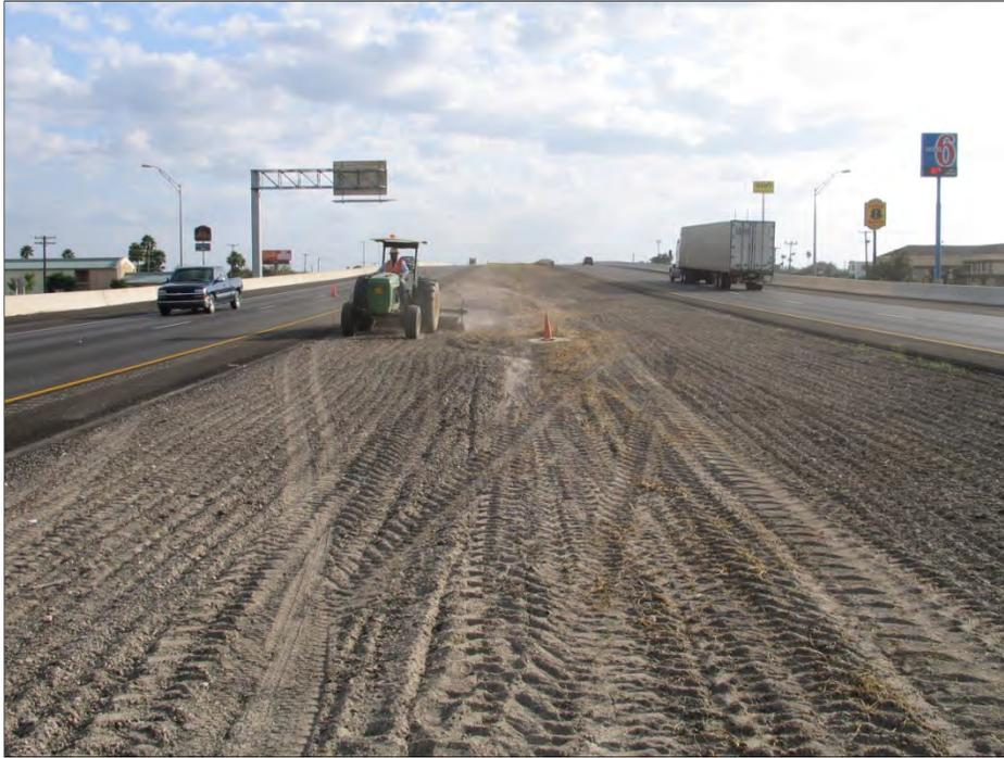
**Figure 1.1. Seeding a Recently Completed Right of Way along US HWY 77 in South Texas.**
