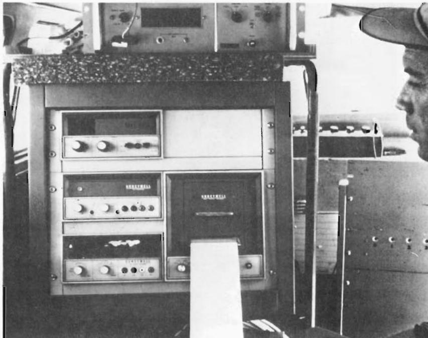
Figure 3.8. Honeywell Data Logging System
