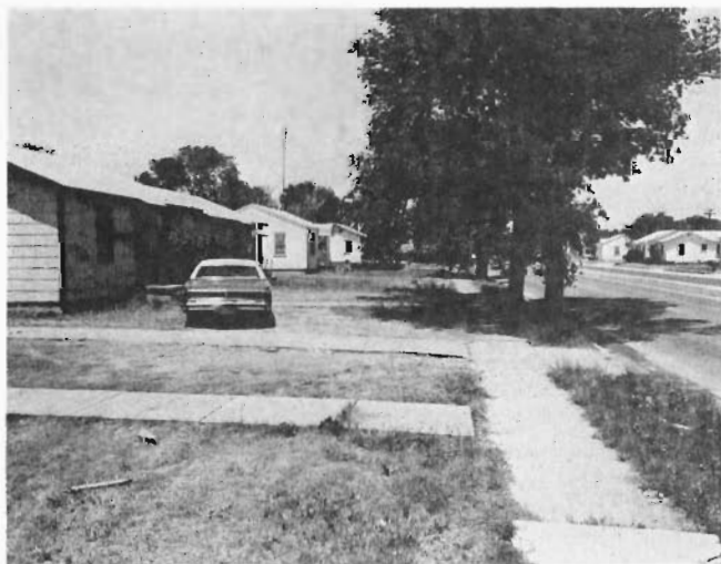
Views of front yards before construction
