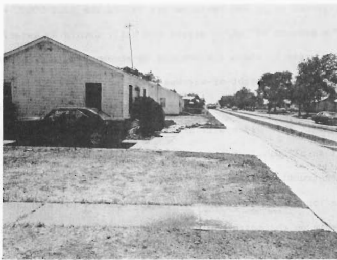
Views of front yards after construction. Curb & Gutter was moved out 13.5' on each side taking trees, sidewalks and requiring new driveways.
