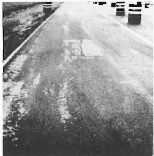
Cracks are developing randomly on this lane under traffic (10/23/87). Station 428+10, offset 13' Lf. CT.
