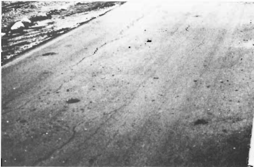
Note longitudinal cracks in wheelpath and center of lane; picture taken at 183 days on Dec. 23, 1987.
