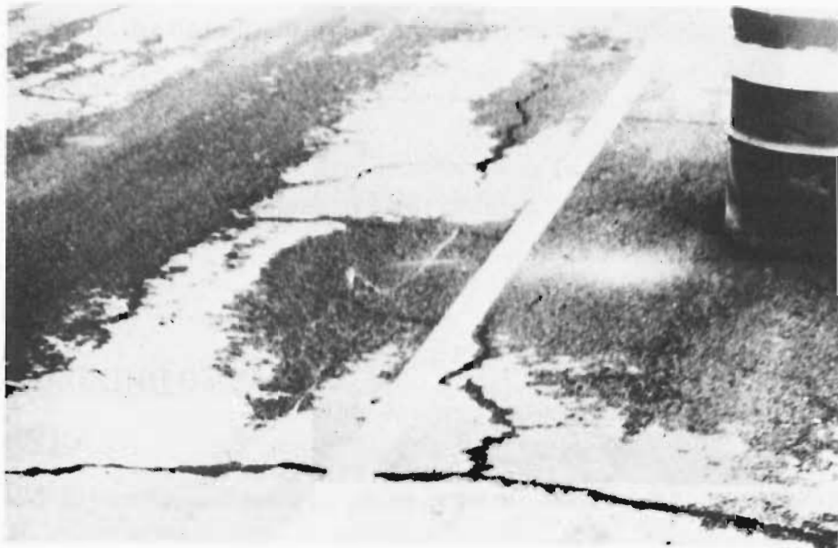
Picture taken at 122 days of alligator cracks. Taken on Oct. 23, 1987 on west lane of SH 146 feeder looking north.
