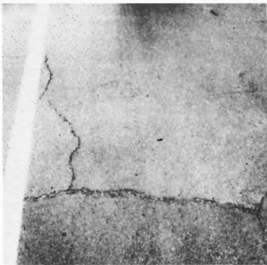
Close-up of alligator crack in area not under traffic. Taken at 122 days (10/23/87). Station 426+53, offset 3' Lf. CT.
