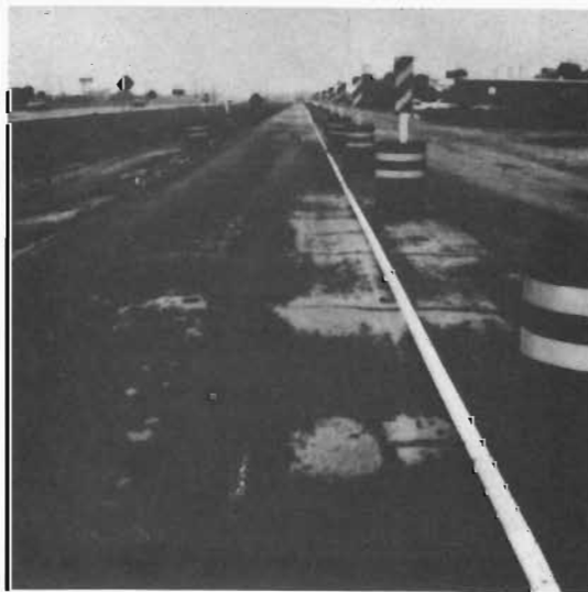
Transverse cracks are shown in this area under traffic on 10-23-87. Station 429+50, offset 2-3' Lf.CT.
