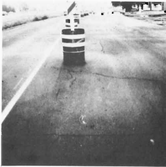
Area not under traffic pictured at 122 days on 10-23-87 showing inter- secting cracks. Station 426+73, offset 3' Lf.CT.
