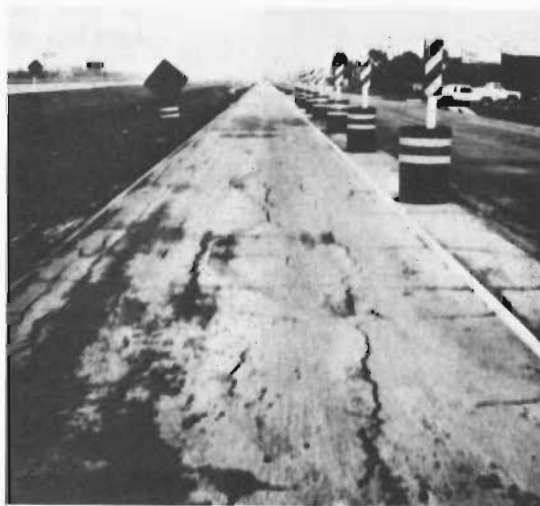
Alligator cracks on lane under traffic at 122 days (10-23-87). Station 431+50 to 433+50 Lf. CT.
