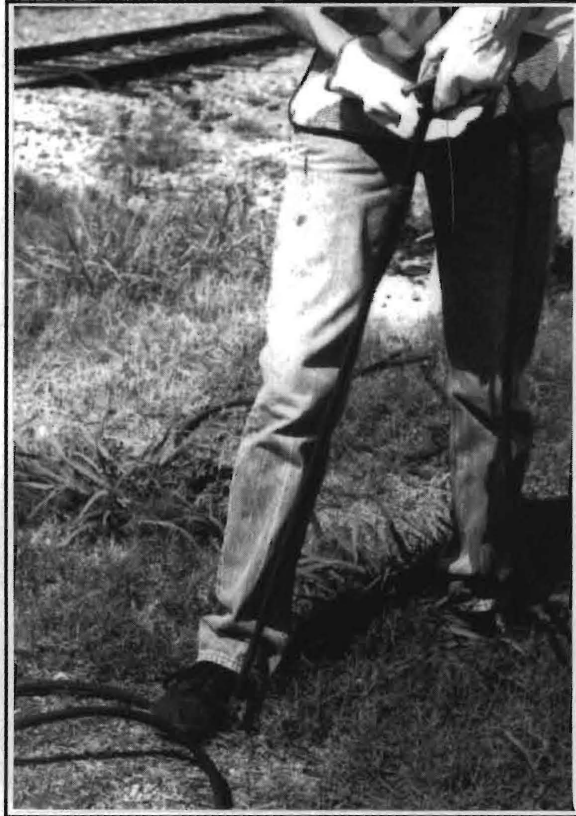
Figure 4-5 Stretching road tube to slide collar toward clamp
