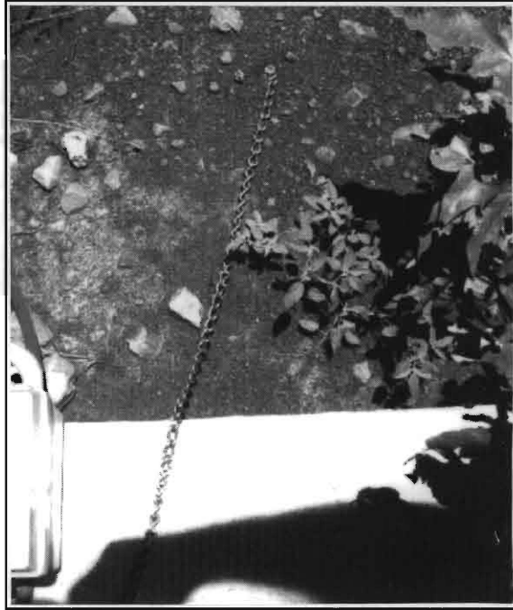
Figure 4-10 Attaching chain to 60d nail in ground when no fixed object is available
