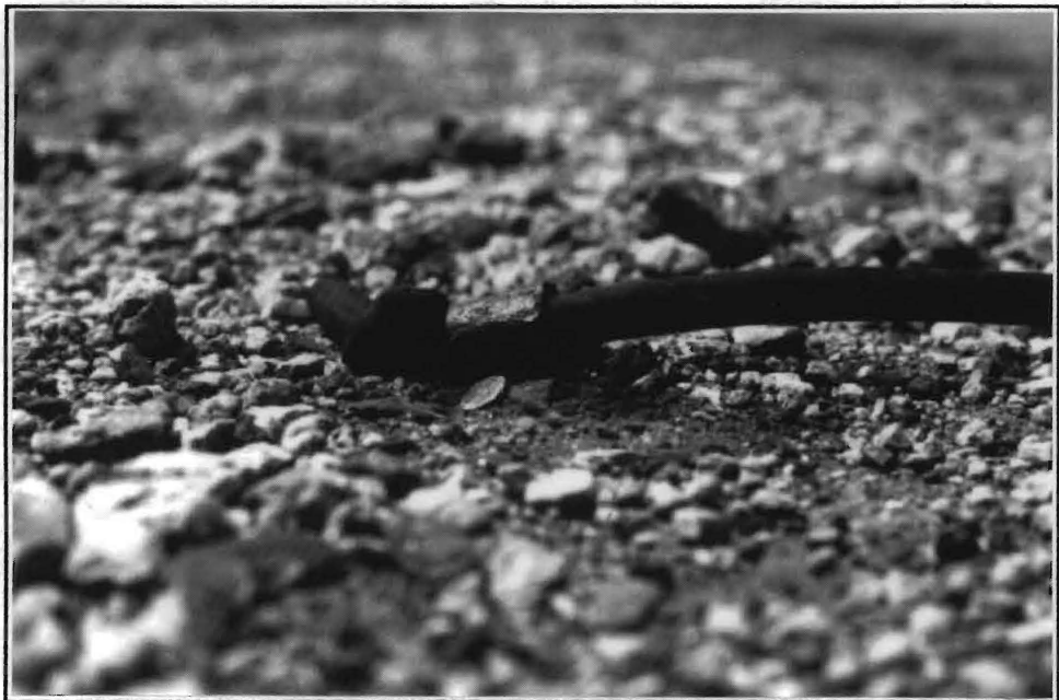
Figure 4-4 Setting clamp nails flush
