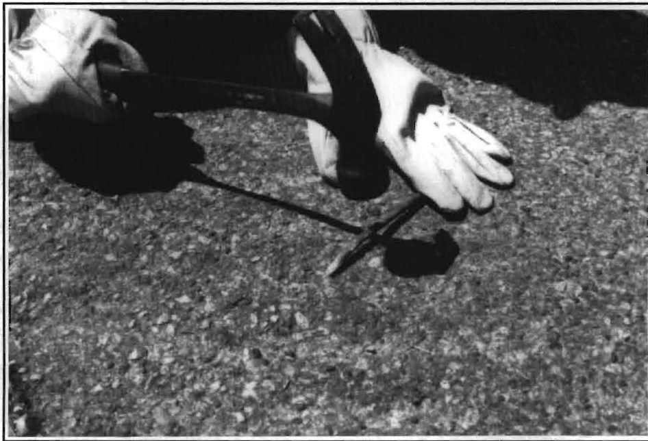
Figure 4-35 Straightening 60d clamp nails for reuse
