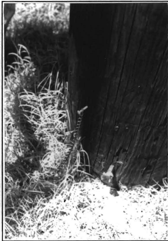
Figure 4-7 Attaching chain to nail in utility post
