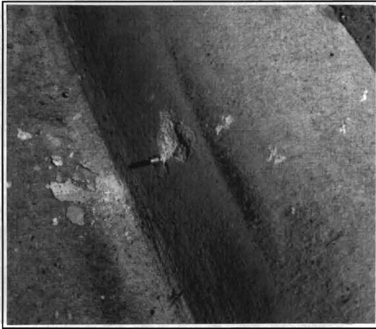
Figure 4-19 Stud in curb side
