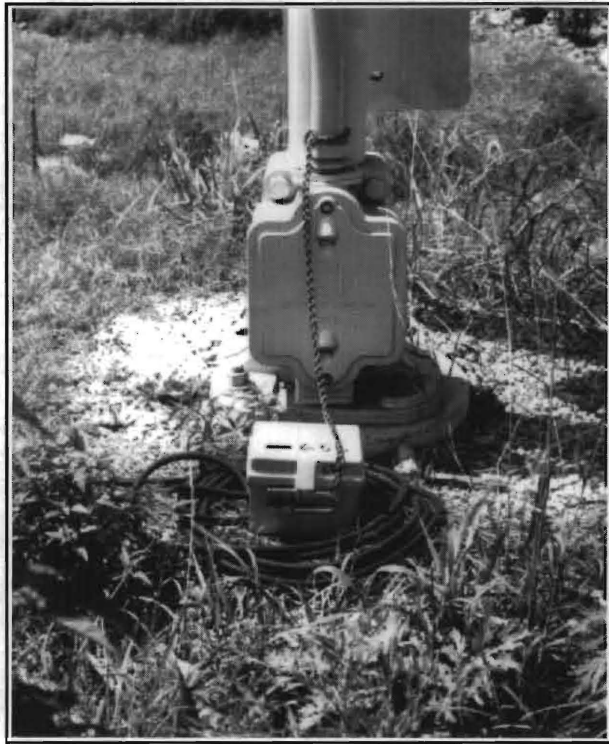
Figure 4-8 Attaching chain to railroad barricade post
