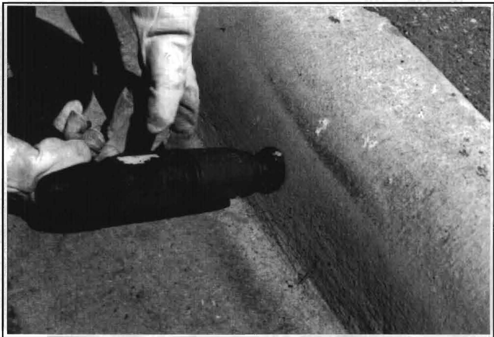
Figure 4-18 Shooting stud into curb side
