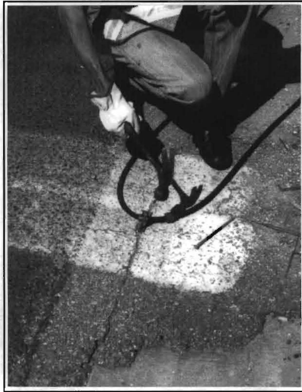
Figure 4-15 Nailing clamp at concrete edge
