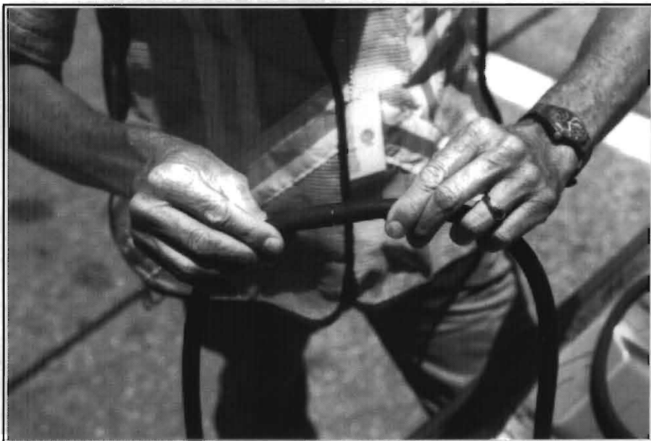
Figure 4-25 Closing rubber tubing over copper extension
