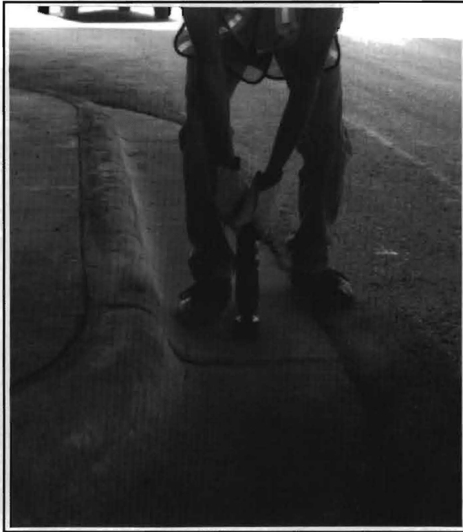
Figure 4-16 Shooting stud into lower curb
