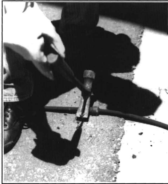
Figure 4-34 Removing clamp nails
