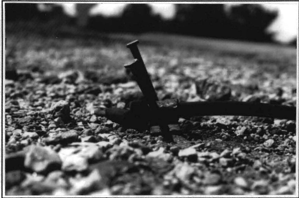
Figure 4-3 Nailing clamp at angle
