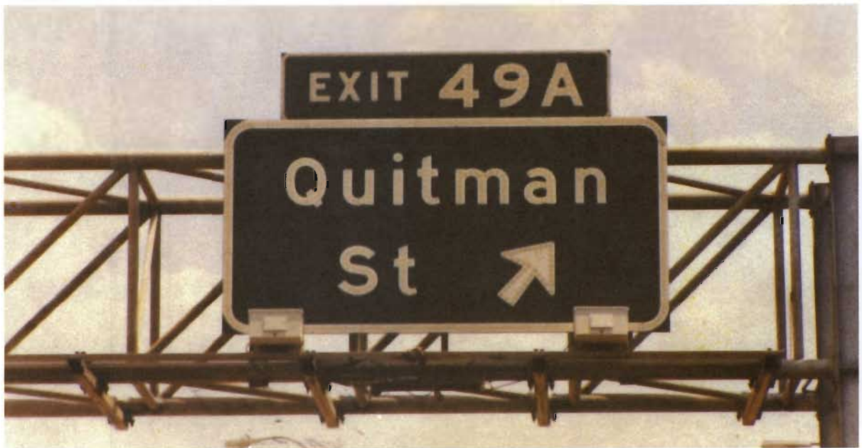
GES-2C Green Sign Paint without Topcoat - 10 Years Field Service Good Condition in regards to Color and Surface Condition
