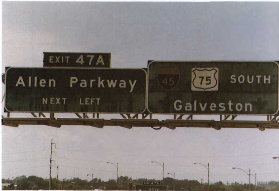
FIGURE 1: Deteriorated Porcelain-enameled Sign in Houston, Texas
