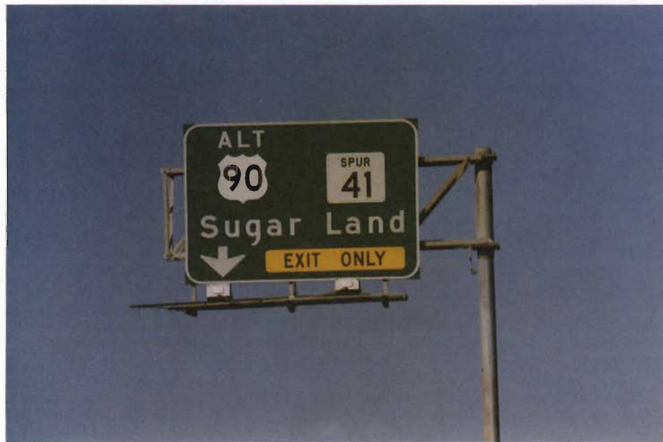
FIGURE 12: Refurbished Sign Panels using High Specific Intensity Reflective Sheeting Applied Directly to the Aluminum Extrusions after 5 Years of service -Good Condition.
