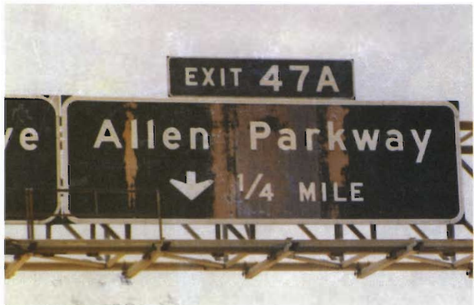
8 years Field Service - The release agent on plastic coated plywood substrate caused delamination. Coating delaminated after 5 years.
