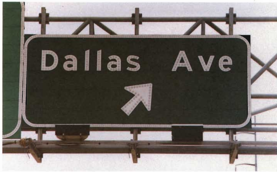
Thermosetting Polyester Coating - Original Condition
