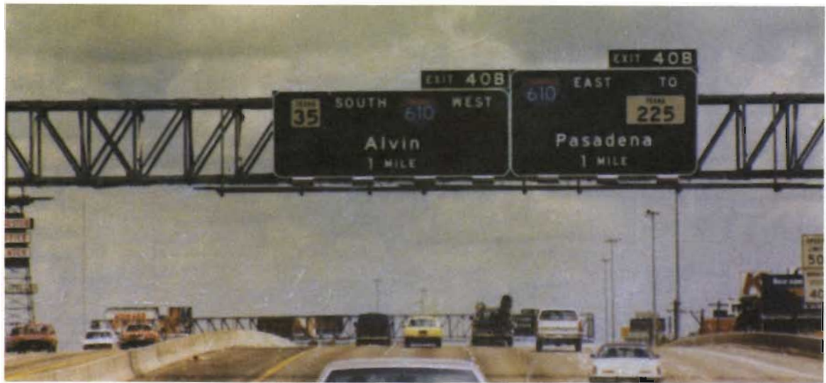
FIGURE 10: Two Thermosetting Polyester Coated Sign Panels that were placed on a contract installation in 1982.
