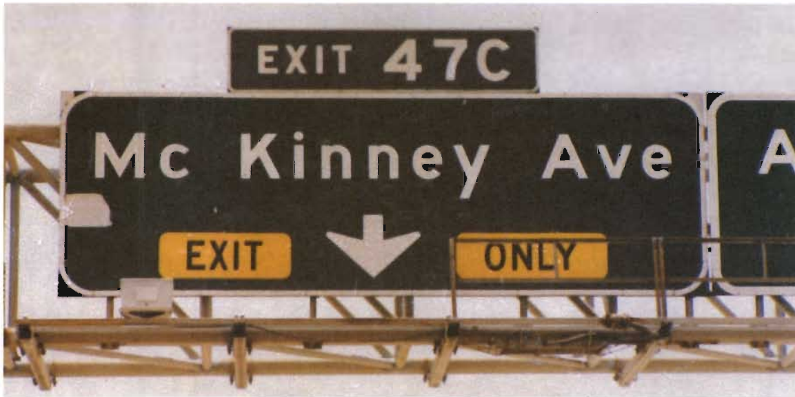
FIGURE 9: Showing Thermosetting Polyester Coating Delamination due to Improper Cleaning of Substrate Prior to Application of Coating
