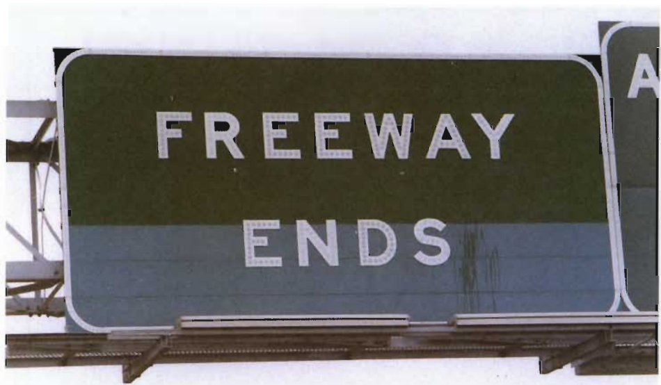
Top extrusions coated with thermosetting polyester. Bottom extrusions coated with polyurethane. Polyurethane faded after two years.
