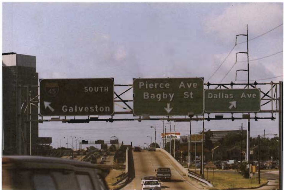
Three different experimental coatings on one structure. From left to right; sign enamel with acrylic top coat, polyurethane, and thermosetting polyester. The acrylic top coat peeled off, but the sign enamel is in good condition.
