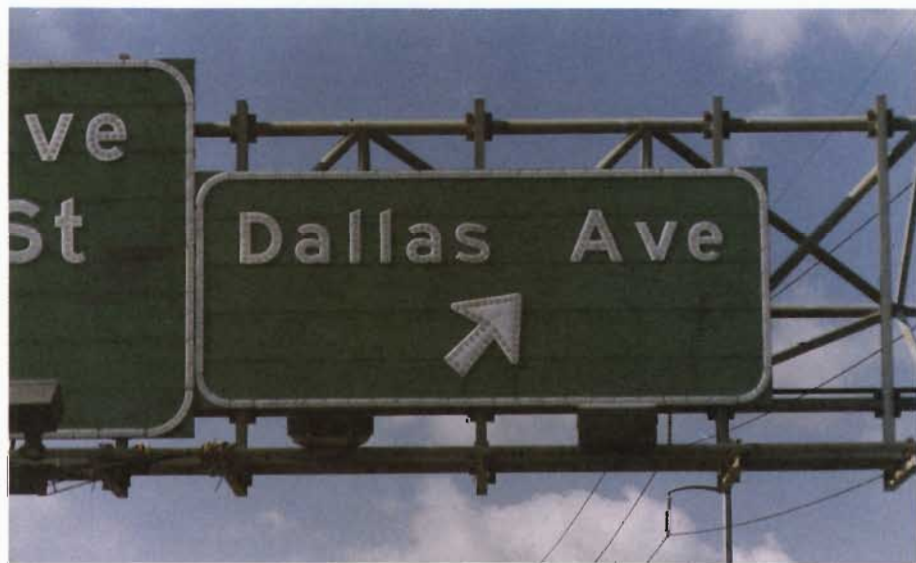
10 Years Field Service - Good Condition in regards to color and surface condition.
