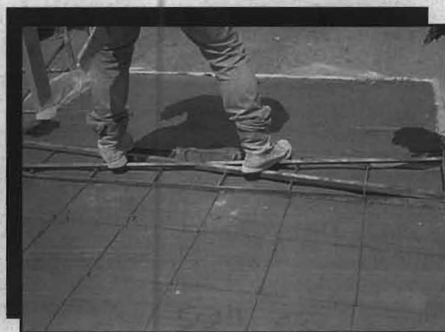
FIG.4: On the job at Rainbow. Left to right from top: barrels of blast waste awaiting S/S treatments; adding blast waste to specially designed mix; pouring the S/S mix (note worker's protective gear); and forming the 12-by-12-by-6-inch blocks.
