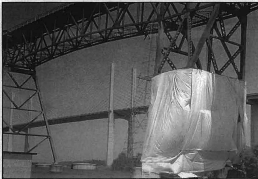
FIGURE 3: Enclosing the Rainbow Bridge for sandblasting.
