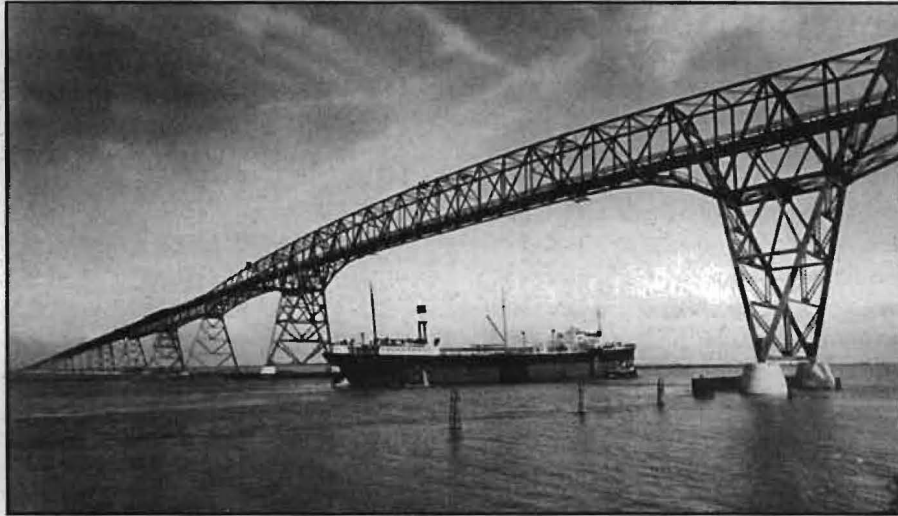
FIG. 2: The Rainbow Bridge soon after completion in 1937. Complex truss work over open water poses a challenge to cost-effective, environmentally responsible rehabilitation.
