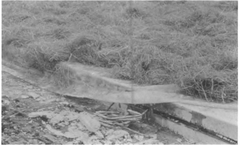
FIGURE 1: Polyethylene sheeting with straw insulation.
