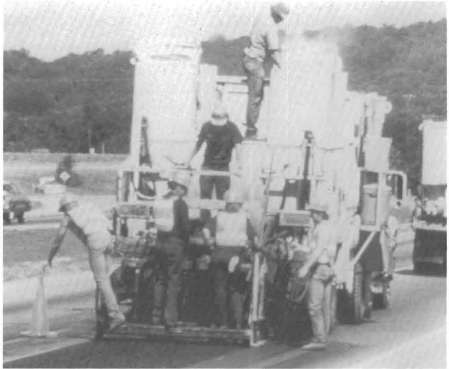
FIGURE 4: A drag box rig used by OKDOT.
