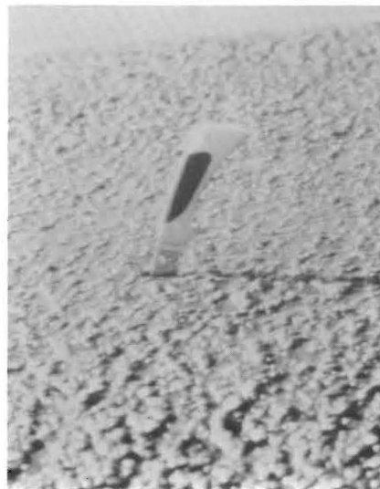
FIG. 1: Polymer-modified slurry seal, prior to breaking.
