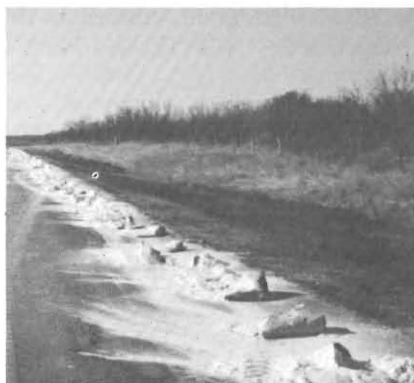
FIG.2 Lime bags spaced 6 feet apart.
