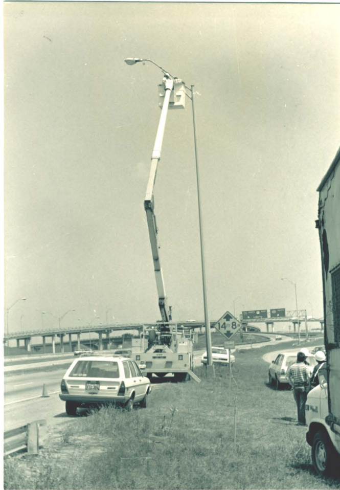
Figure 3 - Site 3 Ramp Luminaire Pole
