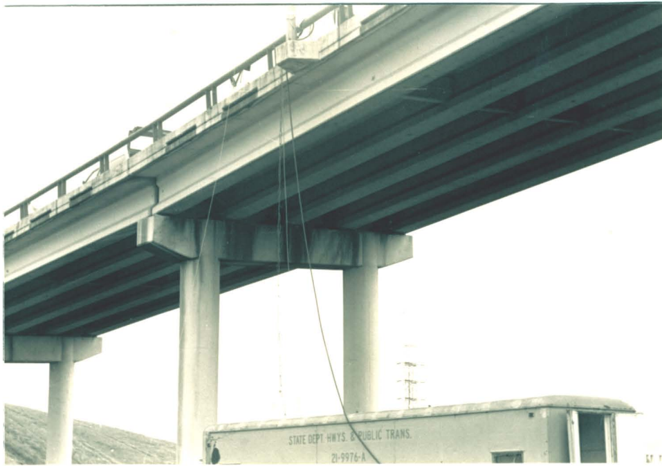
Figure 4 - Site 4 Bridge Ramp
