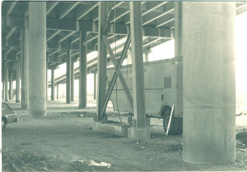
Figure 5 Below Bridge Location
