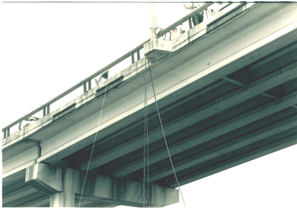
Figure 4.1 Suspended Power and Instrumentation Cables
