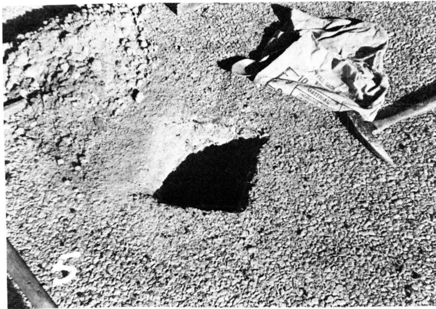
Fig. 2 Sample No. 1 Hole Showing Surface and Base Removed.
