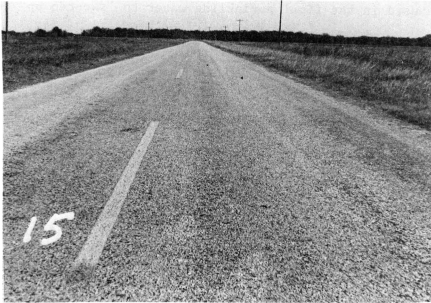
Fig. 6 Roadway Condition at Sample No. 6.
