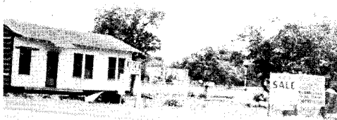
Before new land use can be accomplished in some areas along the expressway, old improvements must be removed.
