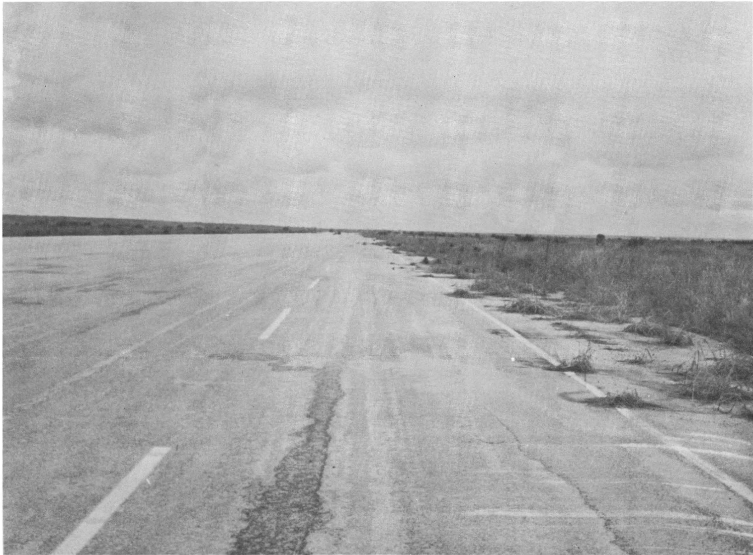
FIGURE 2. DAYTIME VIEW OF SUBJECT CAR LANE
