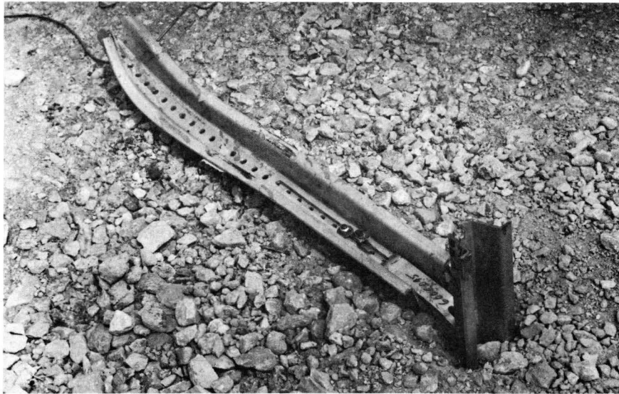
FIGURE 24. EZE-ERECT CONNECTION AFTER TEST 1.
