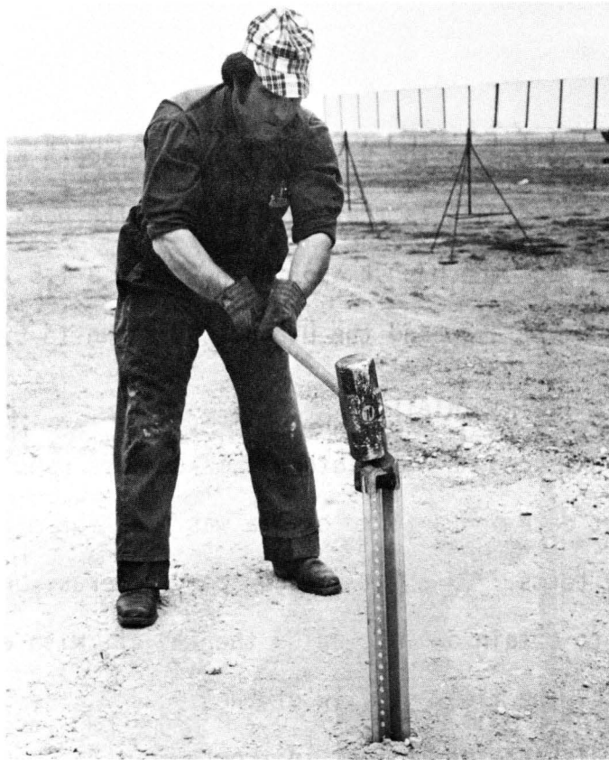
FIGURE 12. DRIVING BASE POST WITH DRIVING CAP.
