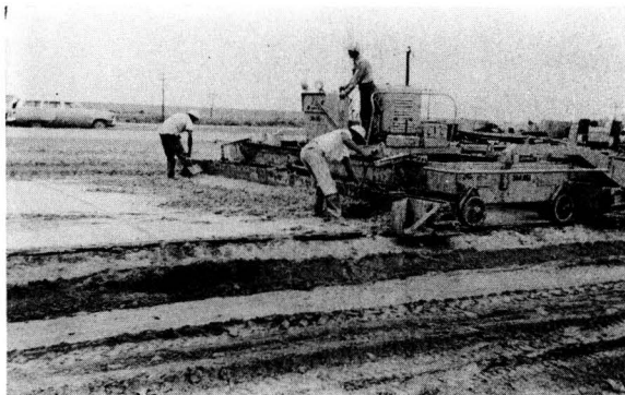
PROPER ATTENTION TO SCREED ENDS AT FORM LINES (p. 74)
