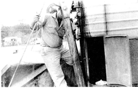
CHECKING ACCURACY OF AIR-ENTRAINING DISPENSER (p. 40)
