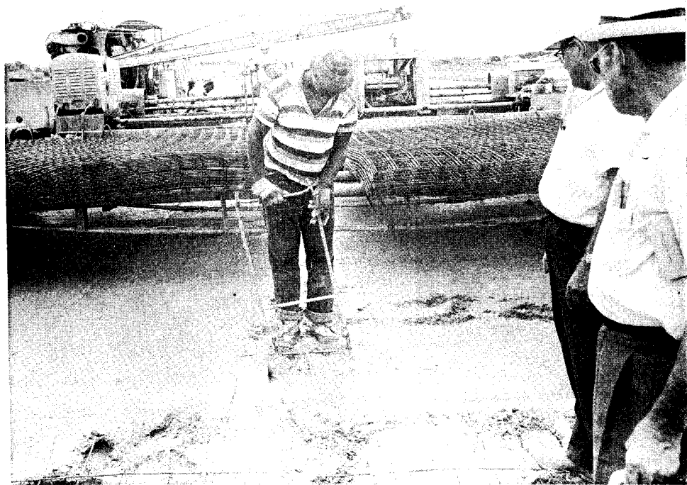
INSTALLING \frac{1}{2} " TIE-BARS IN LONGITUDINAL "CENTER" JOINT
