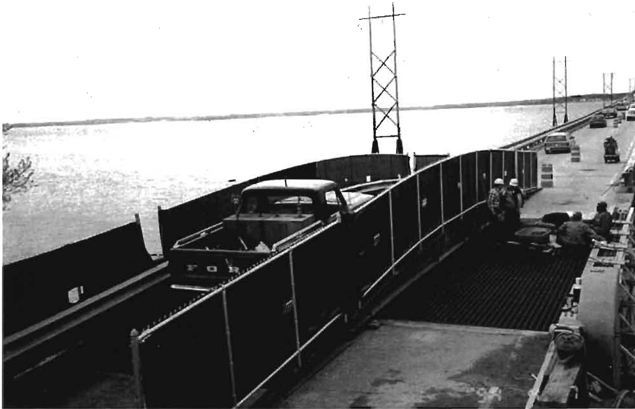
Figure 5.11 Temporary Bridge in Use During Bridge Reconstruction
