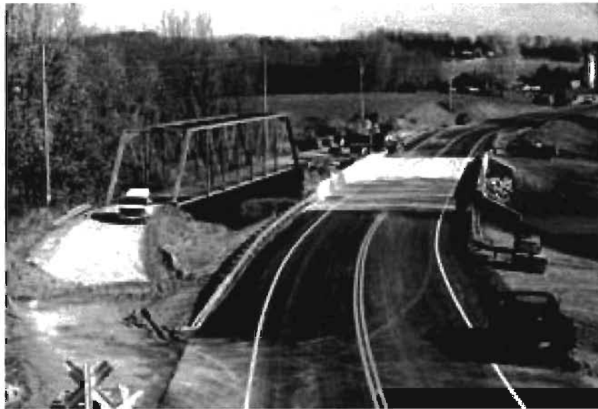
Figure 4.1 Use of a Temporary By-pass Bridge during Bridge Reconstruction
