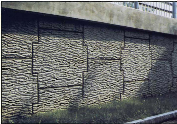
Fractured Granite Reinforced Earth
