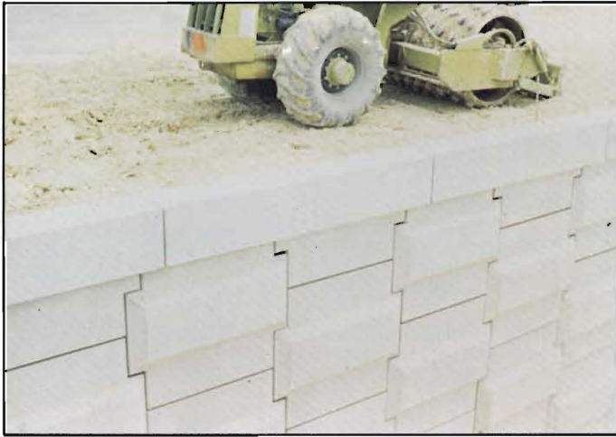
Raised Relief Reinforced Earth
