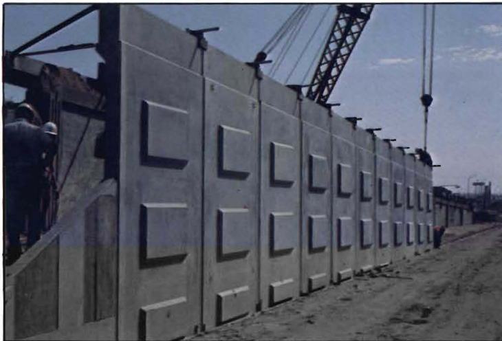
Tensar El Paso, TX US 62 (under construction)
