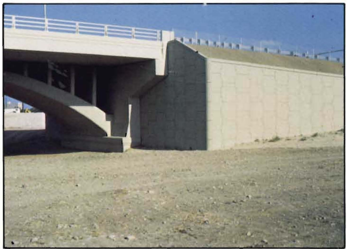
Reinforced Earth Austin, TX Congress Avenue
