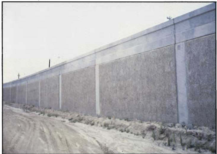
Hilfiker Lufkin, TX Loop 287 (under construction)
