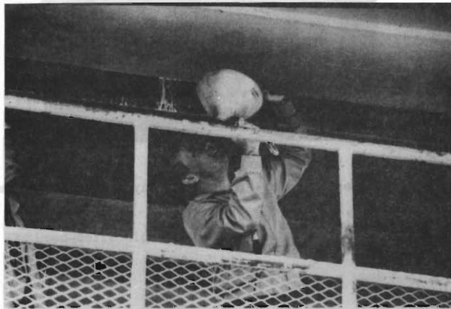
Fig. 22 Detailed inspection of girders for any indication of cracking
