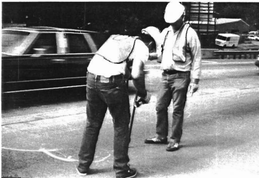
Fig 2.1. Sounding and marking off the delaminated area.
