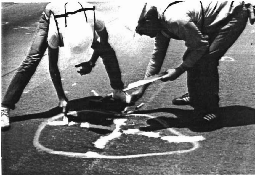
(b) Installation of injection ports.
