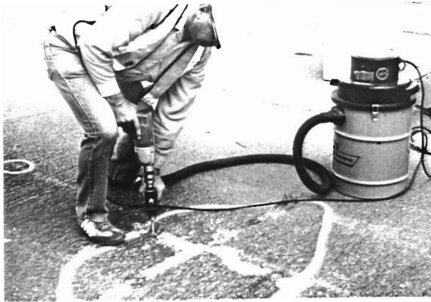
(a) Drilling holes for injection ports.
