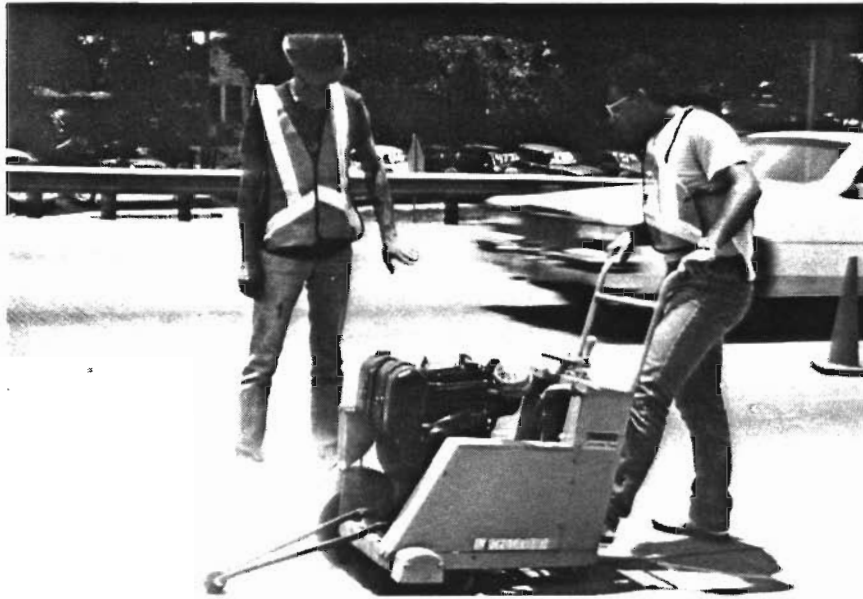
(a) Sawcutting the overlay.
