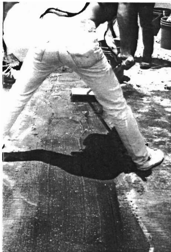
(d) Finishing the surface of the repaired area.
