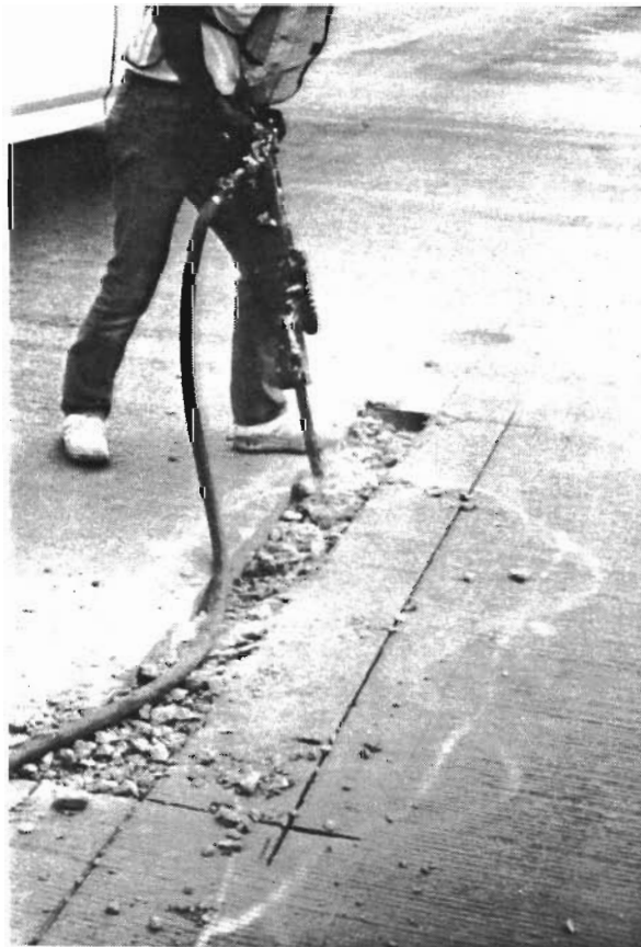
(b) Removing the remaining concrete with a jackhammer.
