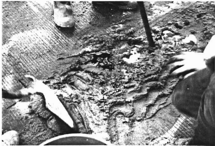
(c) Repair area being filled with polymer concrete.
