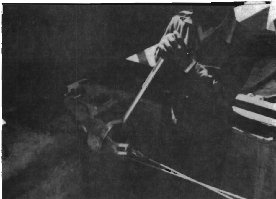
Fig. 5.3 Difficulty involved in exact positioning of wings and coupling of transverse tendon ducts
