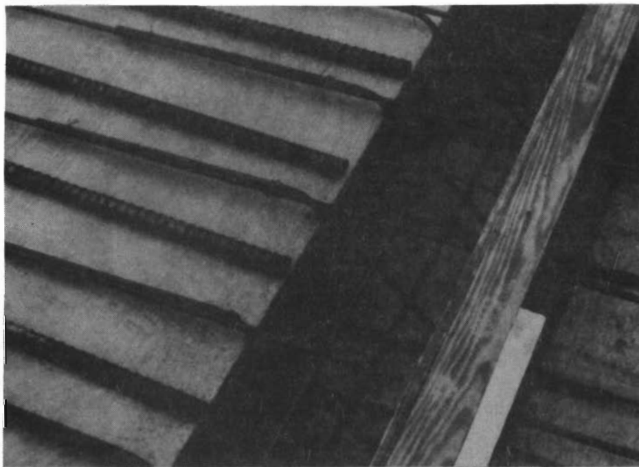
Fig. 2.19 Deck reinforcement cutoff detail over precast panels
