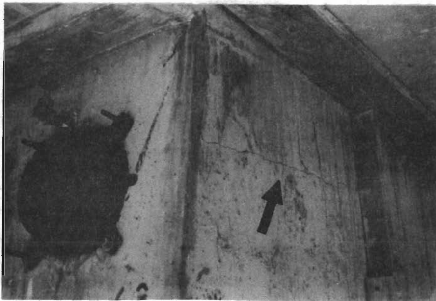
Fig. 4.42 Cracking in anchorage zone of abutment III diaphragm beam (cracks highlighted with black marker)
