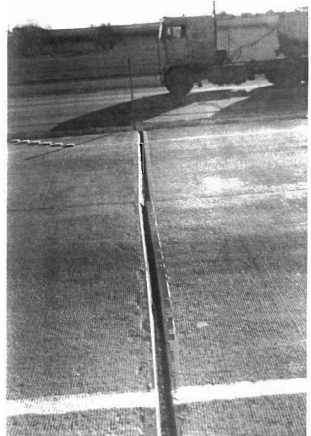
**Fig 3.10.** Open joint between 440-foot slabs.
