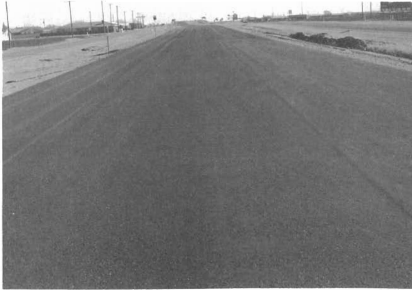
Figure 6 Transverse Rows of Aggregate
