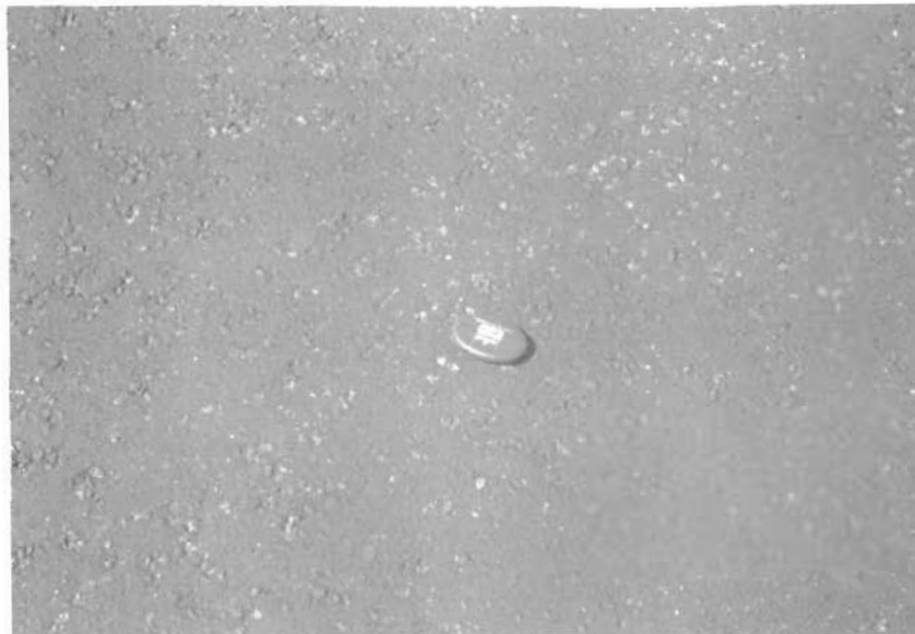
Figure 5 Uneven Aggregate Distribution
