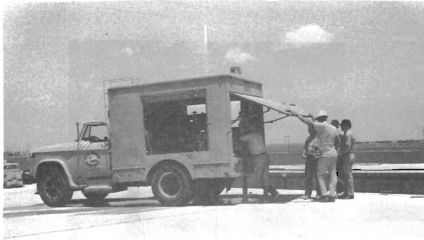
Figure 8. Core Drilling Operations. Drilling Bridge Deck for VSI Specimen
