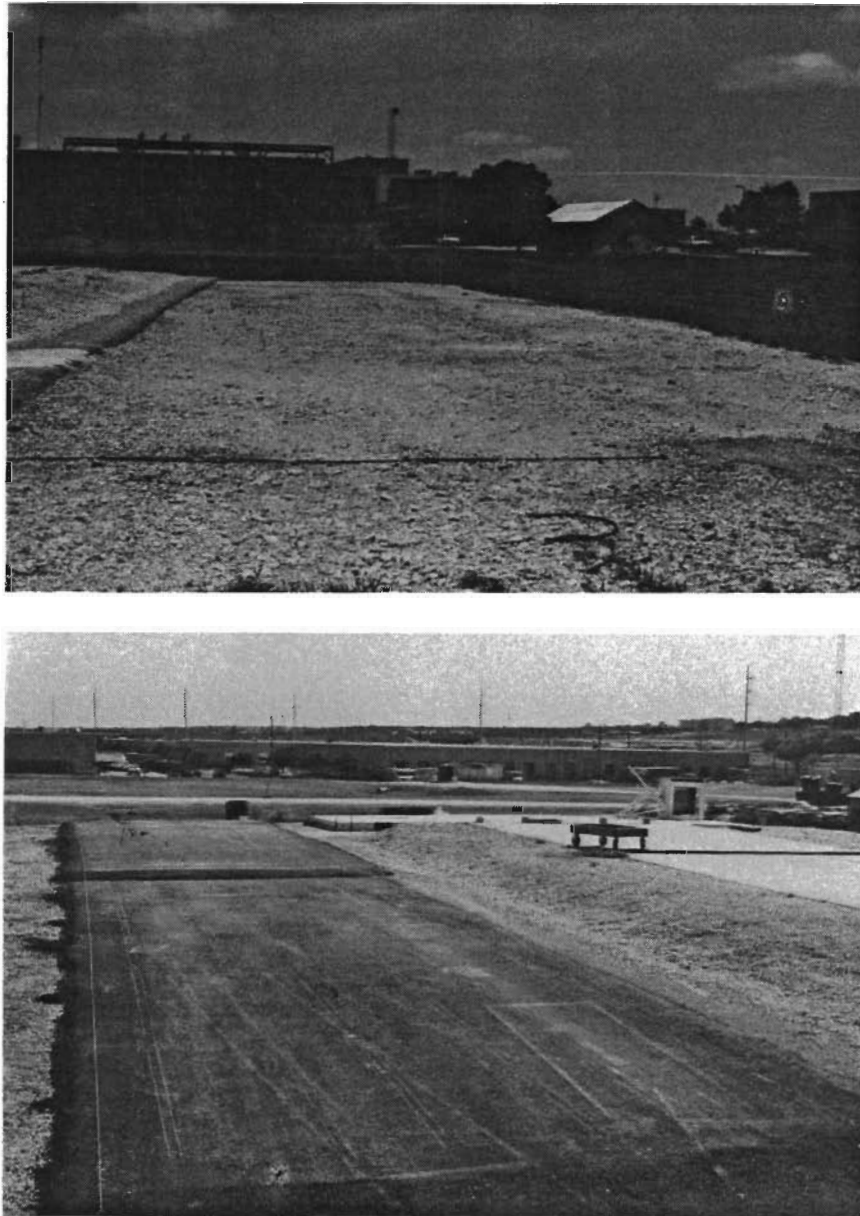
Fig 4.2. Site before and after the asphalt pavement layers were placed.
