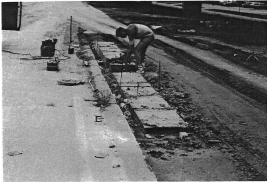
Fig 3.3. Test slabs and instrumentation.
