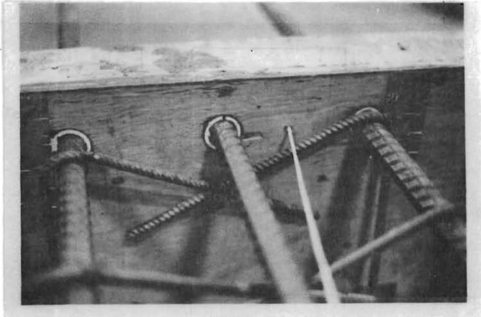
Transverse reinforcement in place prior to casting.
