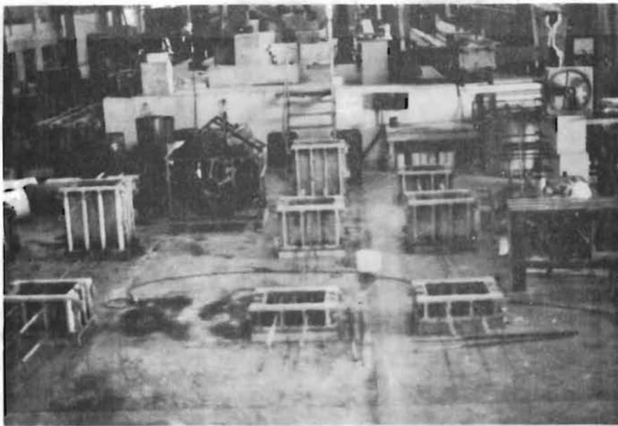
Fig. 2.9 Formwork ready for casting.
