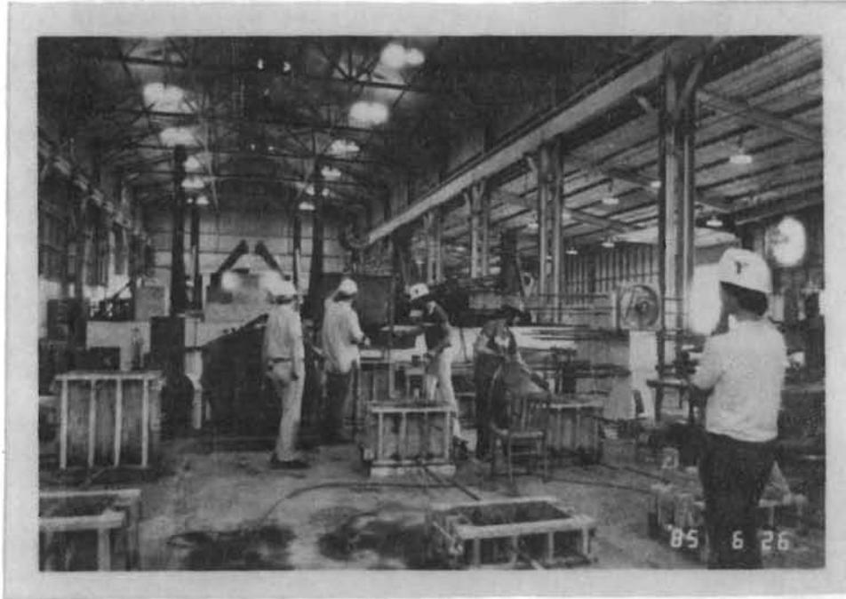
Fig. 2.12 Casting operation - concrete being cast and vibrated.
