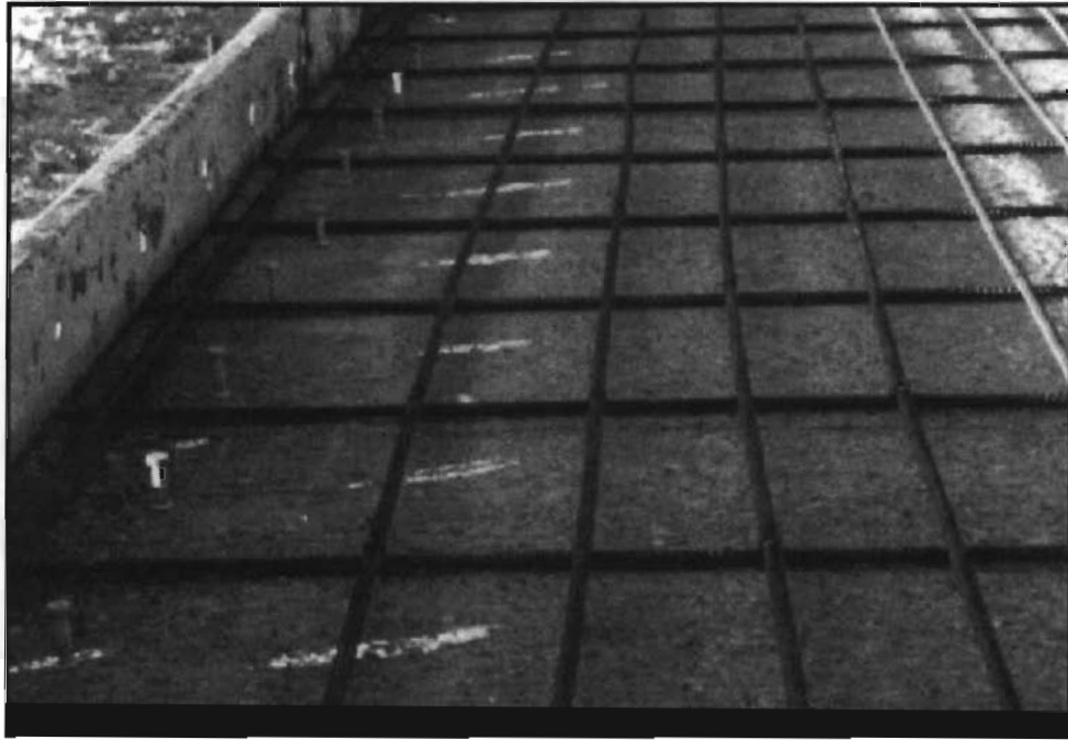
Figure 4.2 Installed shear connectors and reinforcement with formwork
