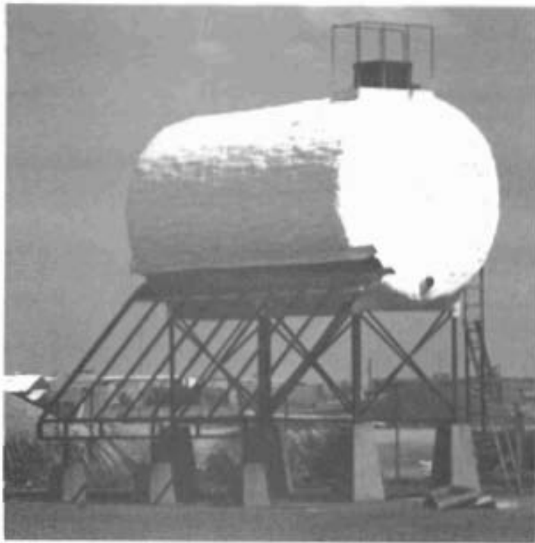
FIGURE 4. Insulated Tank with Collector Racks
