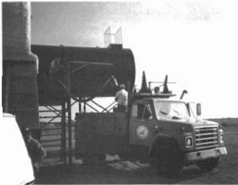
FIGURE 8. Asphalt Being Drained for Use on a Small Job
