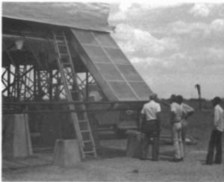
FIGURE 5. Installation of the Collectors
