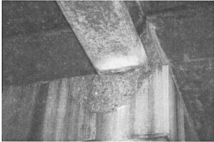
Figure 7.4 Missing bearing pad at I-10 structure
