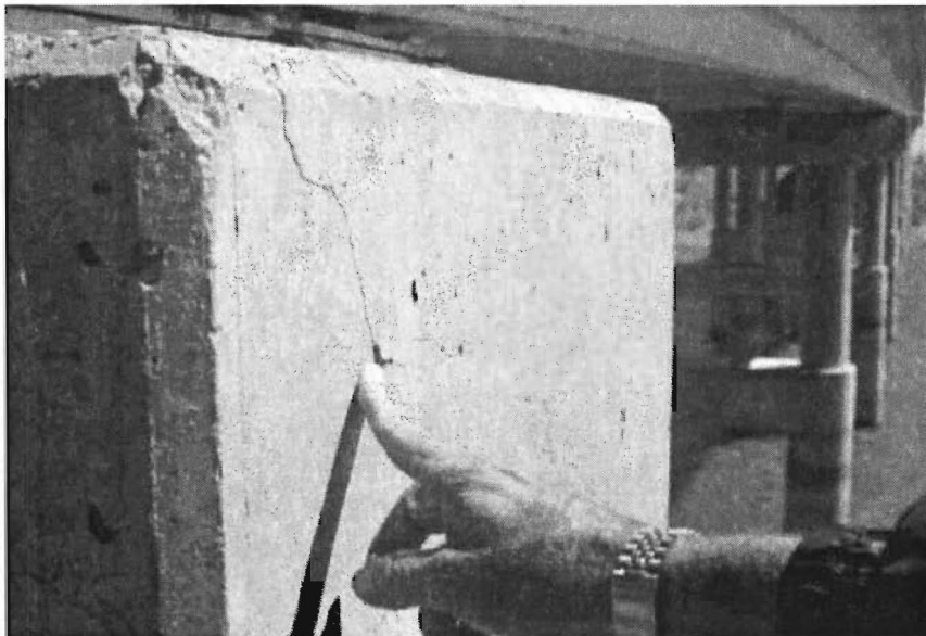
Figure 7.28 Map cracking at ends of bent cap (Bent 5)
