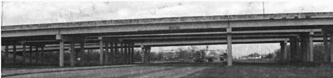
Figure 6.4 Beltway 8 at State Highway 3
