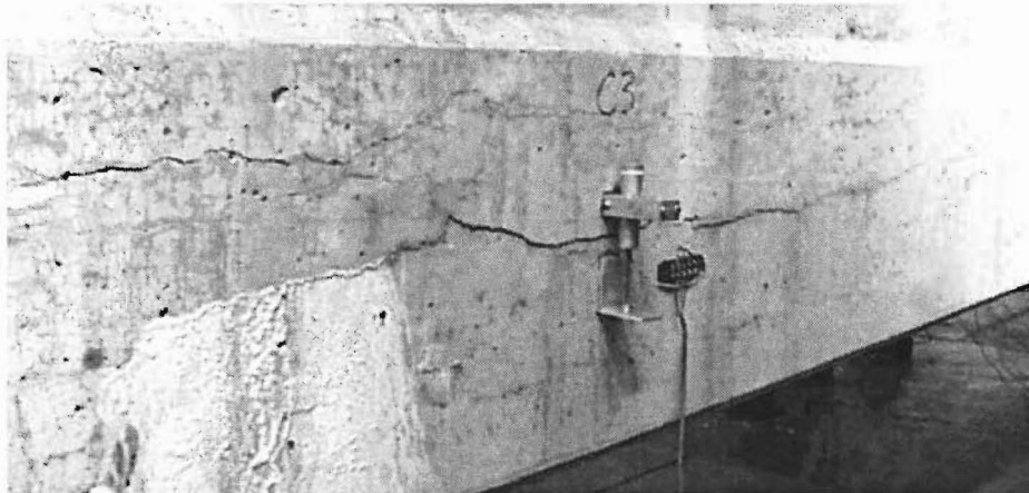
Figure 3.15 Linear potentiometer on west face of BG4F to monitor change in width of pre-existing crack
