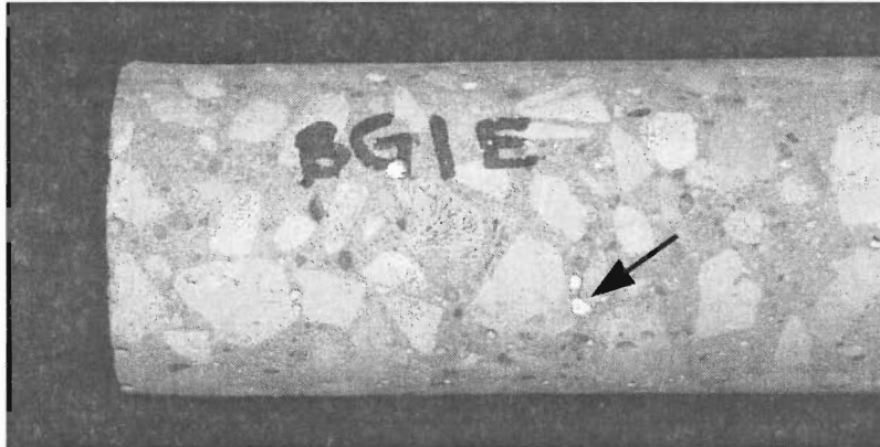
Figure 3.29 White, soap-like substance in voids of core from end-block of BG1
