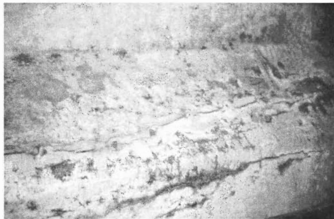
Figure 7.3 Injected sealant on I-10 structure
