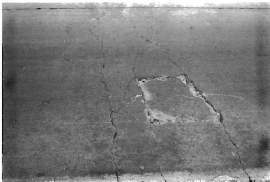
Fig A1.8. Severe punchout.
