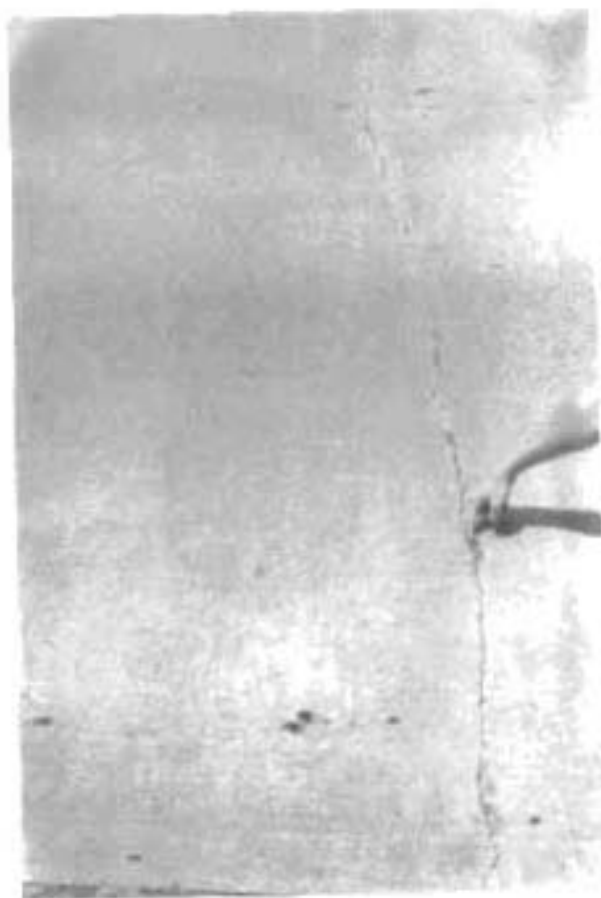
Fig 3A.2 Minor spalling not counted.
