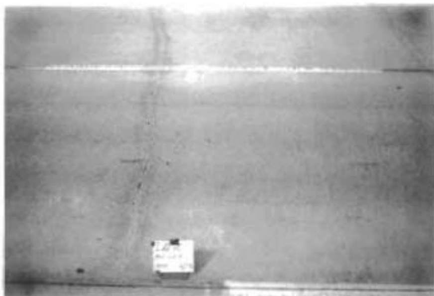
Fig. Al.3. Minor spalling.
