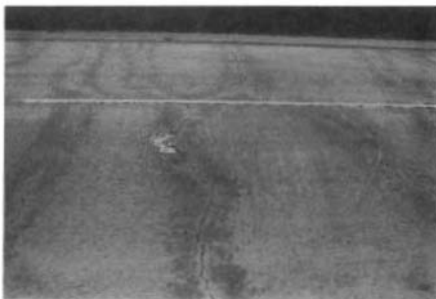
Fig Al.4. Severe spalling.
