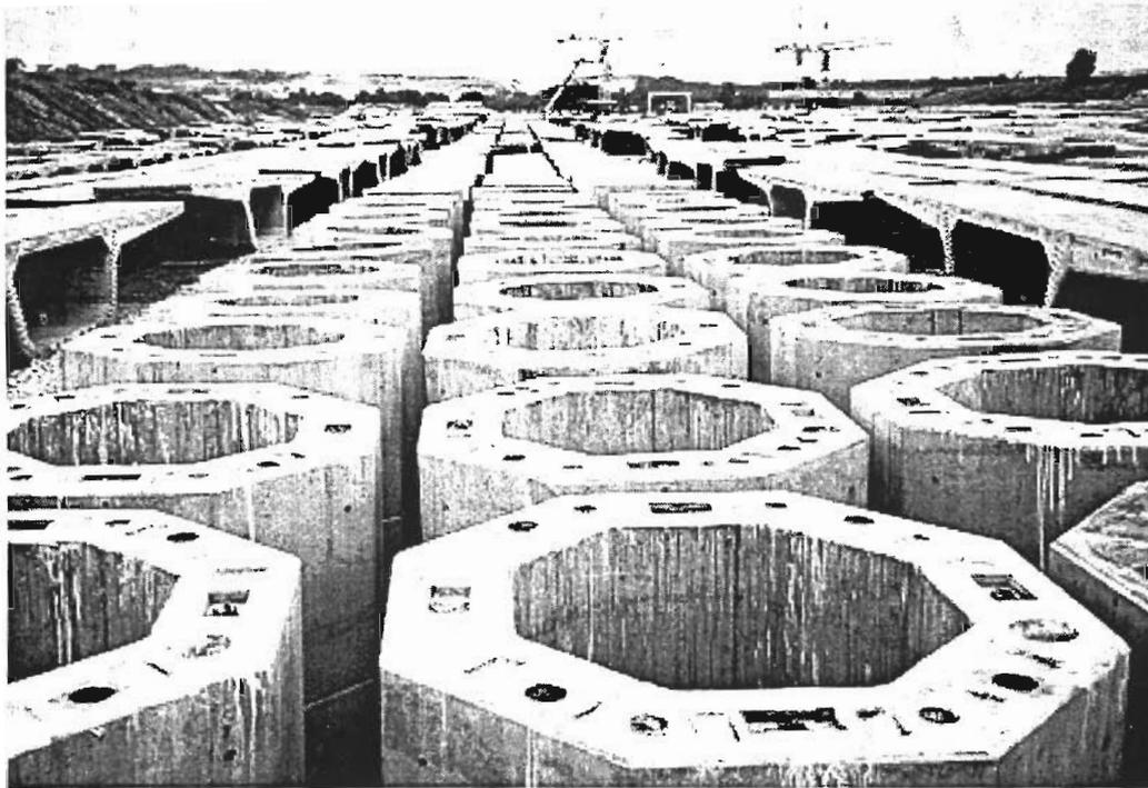
*Figure 4.6 Completed pier segments in storage at the casting yard.*
