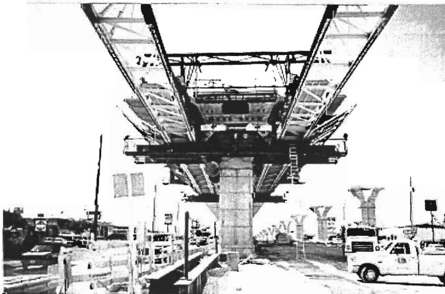
*Figure 4.4 Pier bracket supporting truss.*
