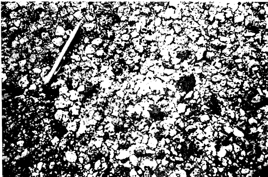
PHOTO 4. CLOSE-UP VIEW OF SURFACE IN PHOTO 3. NOTE THE VESICULAR NATURE OF THE AGGREGATE PARTICLES.
