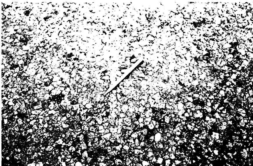
PHOTO 6. A CLOSE-UP OF THE SURFACE FROM PHOTO 5. THOUGH THE SURFACE IS 3 YEARS OLD THE INDIVIDUAL PARTICLES MAINTAIN THEIR SURFACE ROUGHNESS.
