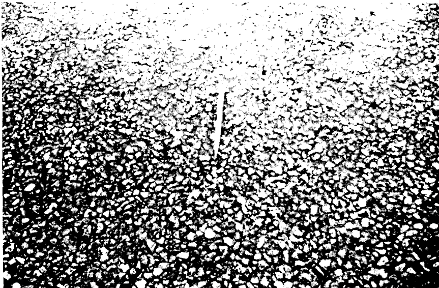
PHOTO 13. CLOSE-UP OF TEXTURE SHOWN IN PHOTO 12. EXCESSIVE EMBEDMENT LEAVES FEW PARTICLES IN BOLD POSITION SUBJECT TO EARLY POLISHING.
