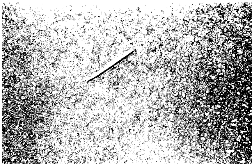
PHOTO 2. CLOSE-UP VIEW OF WHEEL PATH SURFACE FROM PHOTO 1. NOTE LACK OF RUGOSITY OF SURFACE.
