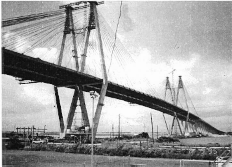
Figure 1-1 Houston Ship Channel Crossing
