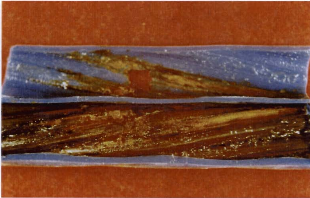
Figure 8- 37 Corrosion under sheathing
