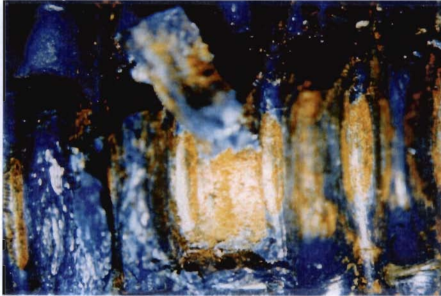
Figure 8- 31 Corrosion under epoxy coating between tooth marks
