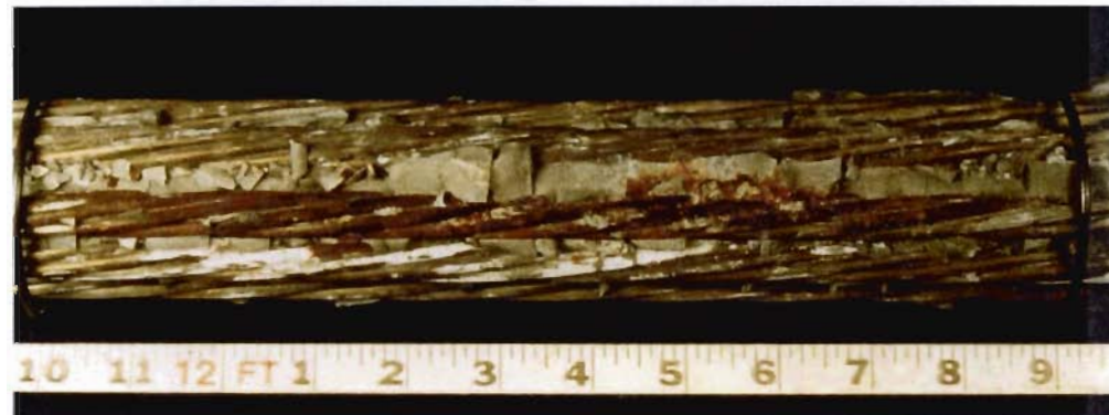
(c) Corroded strands uncovered during post-mortem examination
