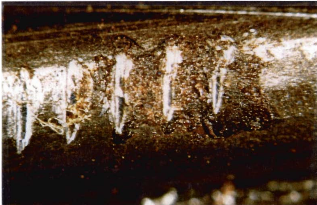
Figure 8- 25 Corrosion between tooth marks on strand
