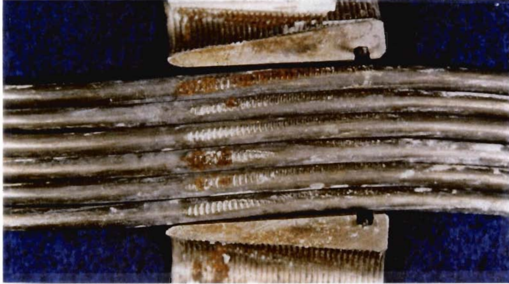
Figure 8- 24 Corrosion at the interface between the strand and wedge
