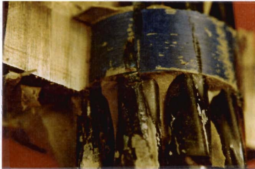
Figure 8- 32 Epoxy coating damaged by contact with deviator ring
