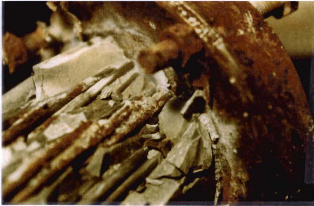
Figure 8- 26 Corrosion of strand adjacent to deviator ring
